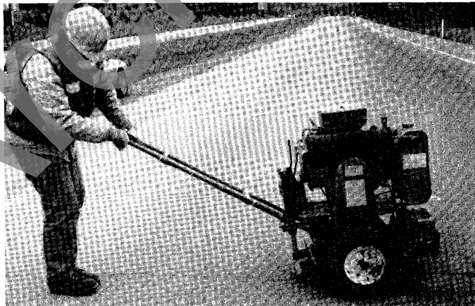
Figure 5-5. Routing with a rotary-impact router.
