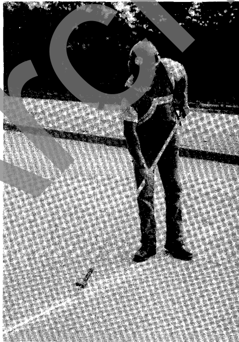
Figure 3-7. Adjustable backer rod insertion tool.
