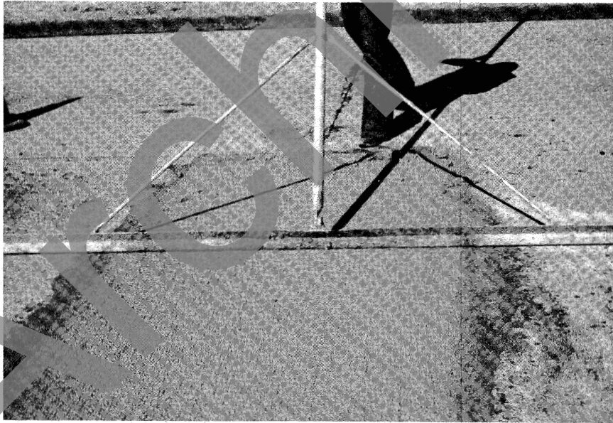
FIGURE 21 – FINISH CONCRETE Occasionally, additional floating is required to provide a level patch.
