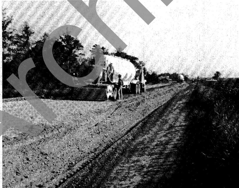
Figure 12. Bulk application using transport with pneumatic pump and mechanical spreader.
