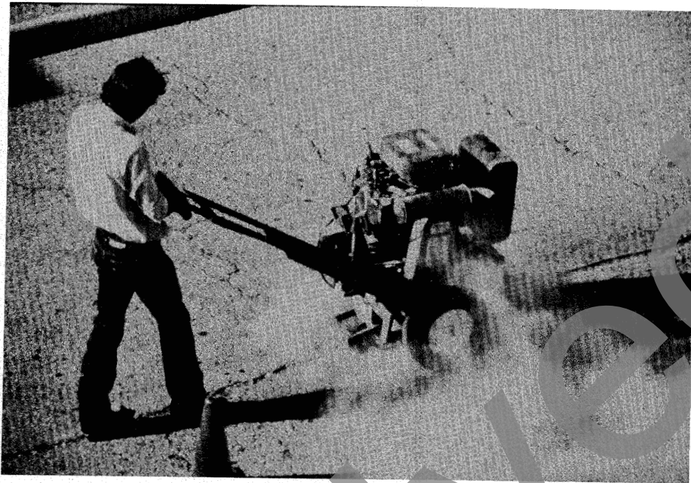
Figure 41. Router for shaping cracks.
