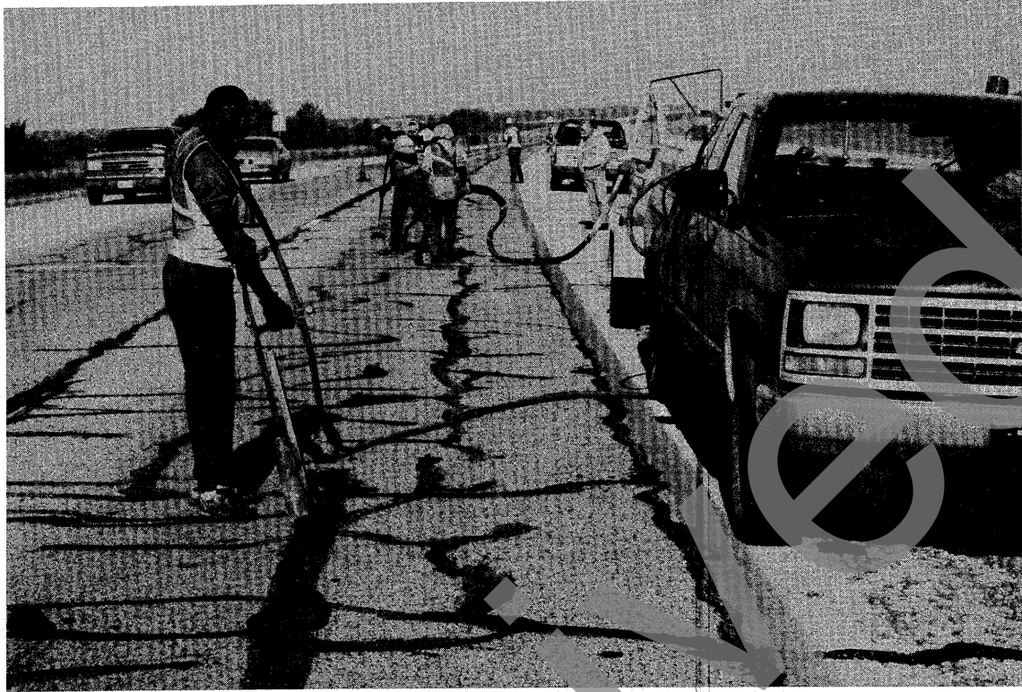
Figure 43. An asphalt kettle with pressure applicator.
