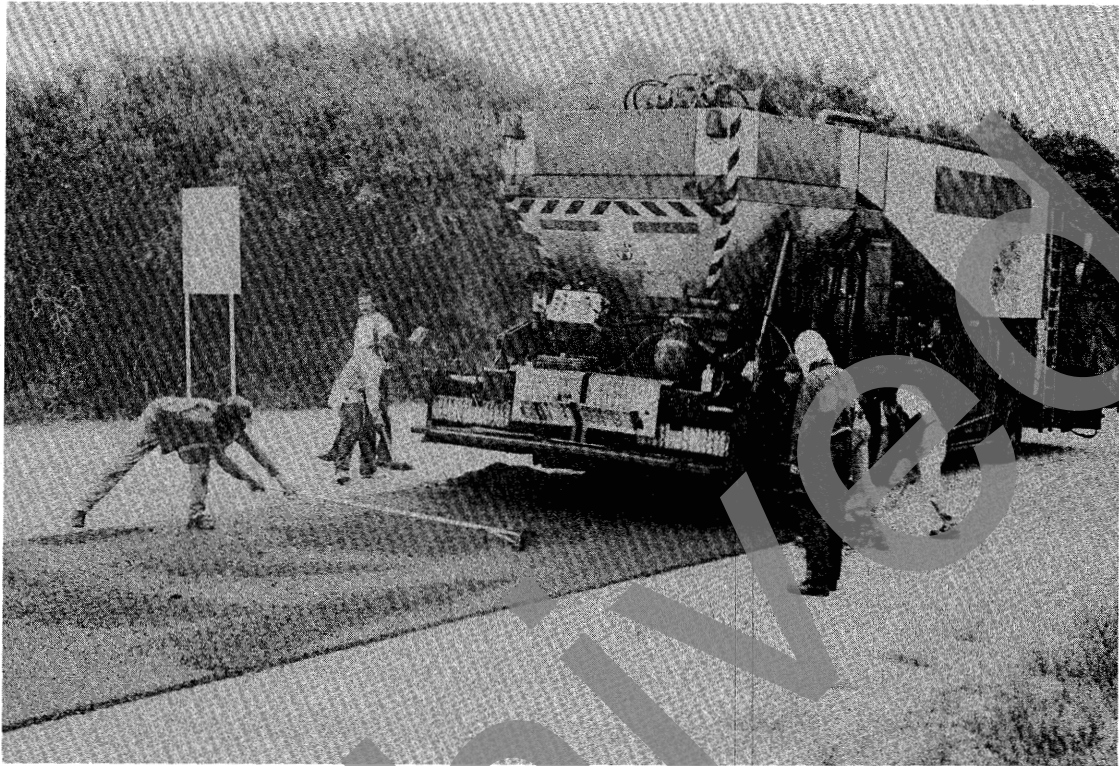
Figure 35. The Novachip paver.
