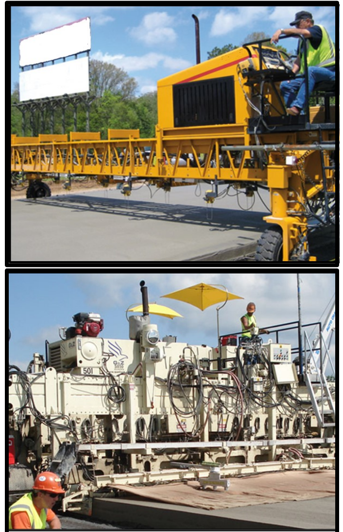
Figure 4. Real-time smoothness measurement equipment for concrete pavements. (Image source: GOMACO, AMES)
