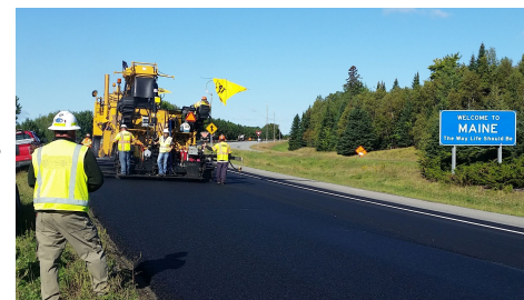
PMTP on I-95 in Houlton, ME. Photo: MaineDOT
