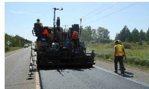
PMTP scans a highway paving job in Minnesota. Photo: MnDOT
