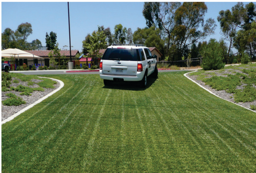
Figure 6-15. Vegetated pavement (photo courtesy of Soil Retention Products, Inc.).
