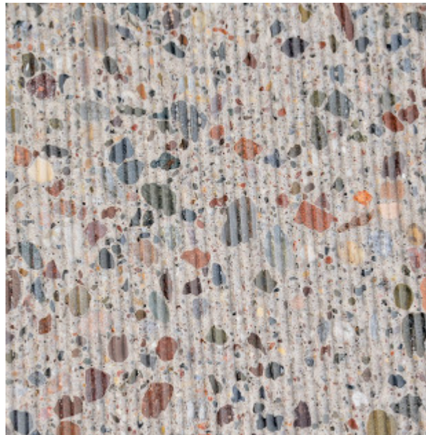
Figure 6-25. Diamond ground concrete pavement surface.
