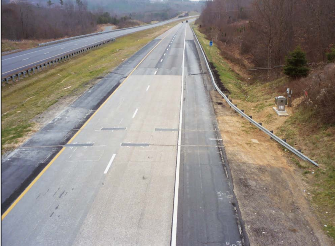
Figure 7. Photo. Two-lane WIM site, with Portland cement concrete (PCC) pavement installed for approach and departure.
