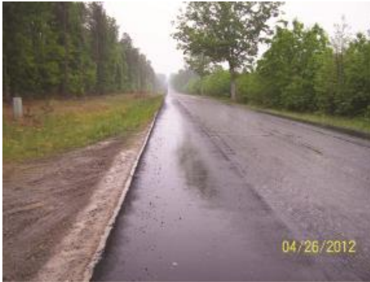
FIGURE E-10 OVERALL VIEW OF ROADWAY FACING EAST
