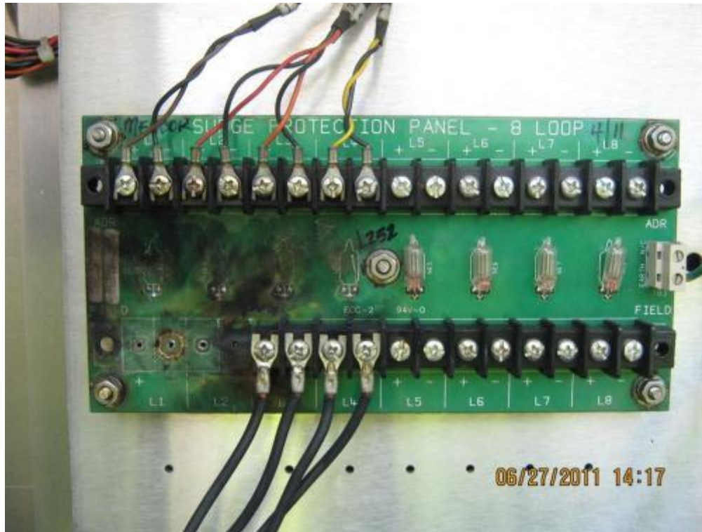
FIGURE F-10 LOOP FIELD CONNECTIONS DESTROYED BY LIGHTNING INDUCED SURGE
