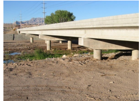
Figure 4: New Beaver Dam Wash Bridge. Source: Mohave County
