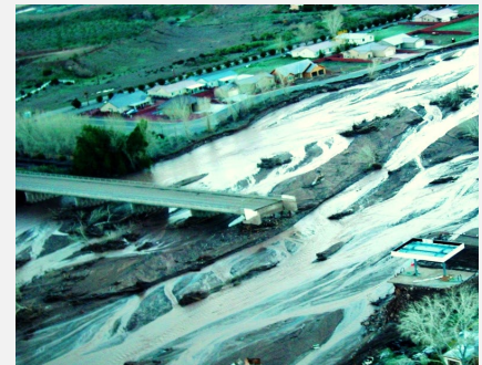
Figure 1: Damage to the Beaver Dam Wash Bridge following heavy floods in January 2005. Source: Mohave County
