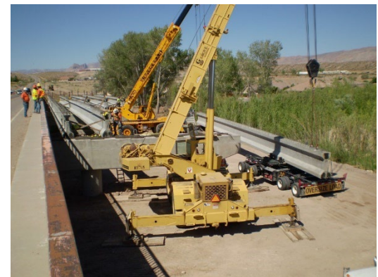
Figure 3: Construction of the new Beaver Dam Wash Bridge. Source: Mohave County
