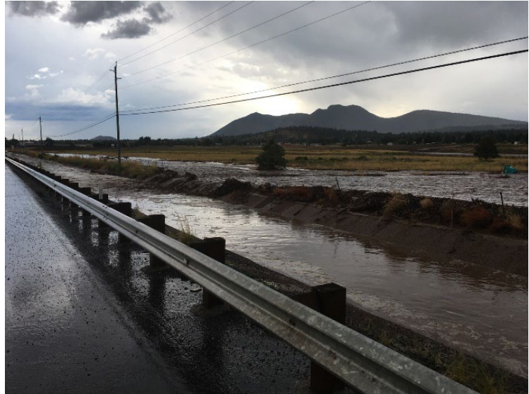
Figure 3: In 2018, the new concrete lined channels along US 89 directed floodwaters to the detention basin and protected the roadway and surrounding homes from major damage. Source: FHWA
