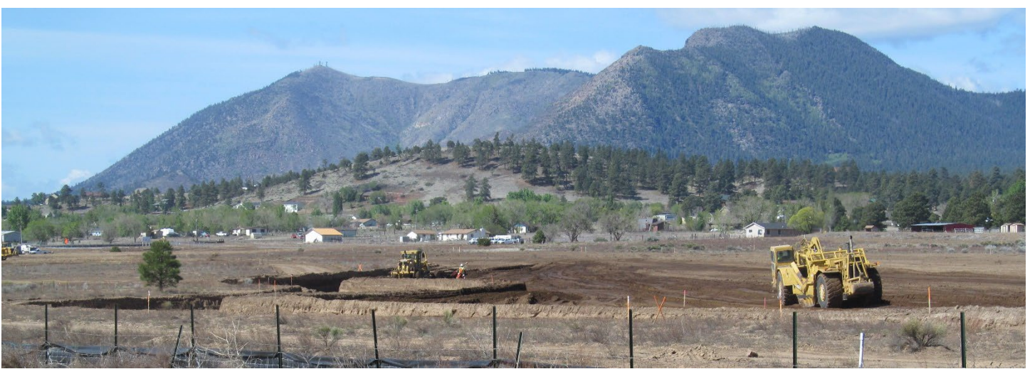
Figure 2: Construction of the detention basin. Source: FHWA
