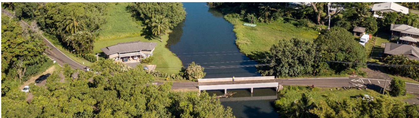
Figure 2: Aerial view of the rehabilitated Wai'oli bridge. Source: HDOT
