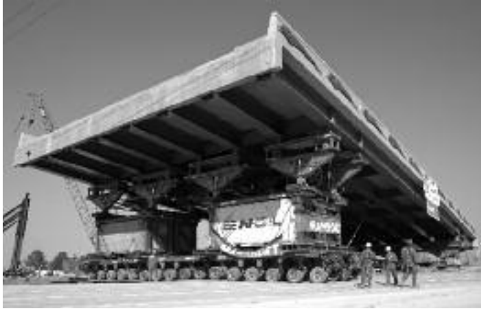
Utah's accelerated bridge construction projects include the 4500 South bridge in Salt Lake City. The prefabricated superstructure was installed using self-propelled modular transporters.
