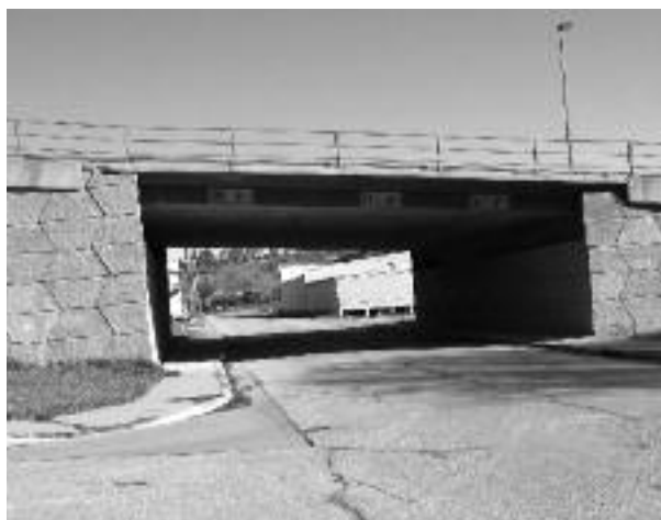
Bridge abutment walls in Warm Springs, SD.
