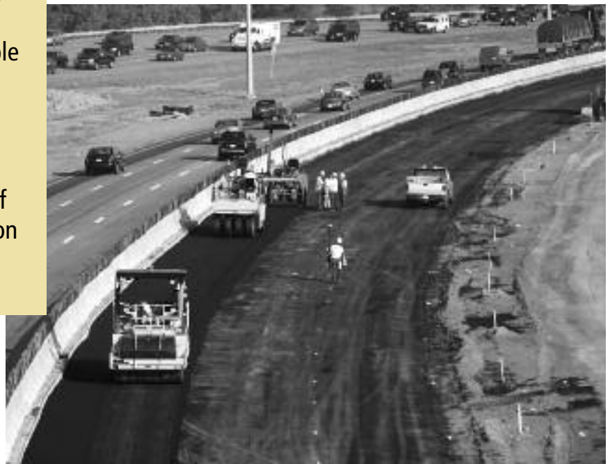
Using transportation asset management and information from management systems, agencies aim to provide the best return for each dollar invested in transportation infrastructure.
