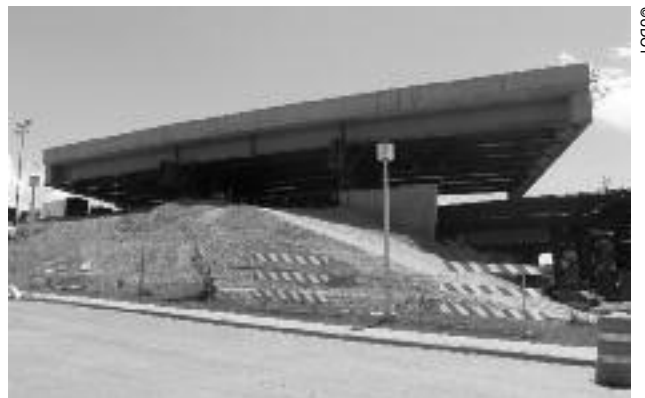
Innovations implemented across the country include the Utah Department of Transportation’s use of accelerated construction techniques for bridges, such as for this bridge on I-80 in Salt Lake City.
