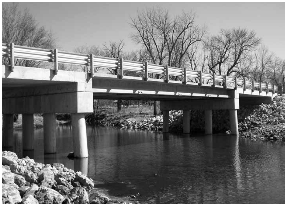
Ultra-high performance concrete pi-girders were used in the construction of the Jakway Park Bridge in Buchanan County, Iowa.
