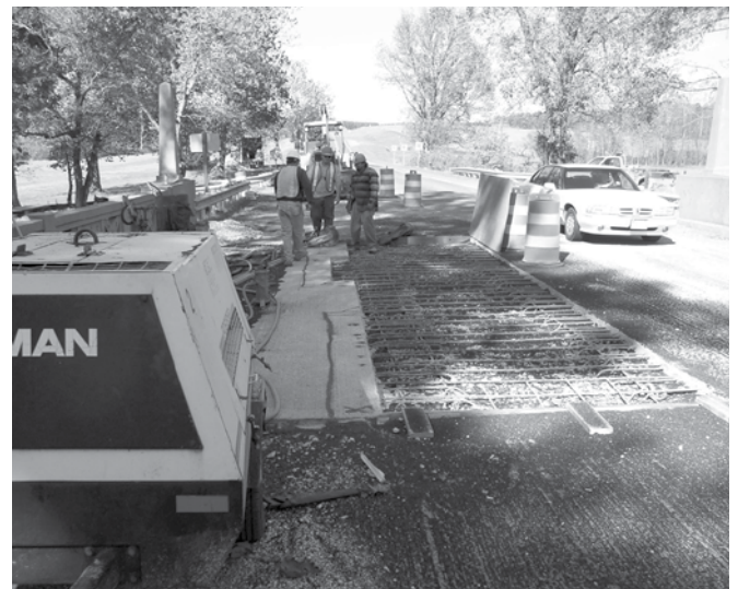
Bridge deck repairs are performed prior to installation of a deck overlay, which can reduce the impact of aging and weathering.
