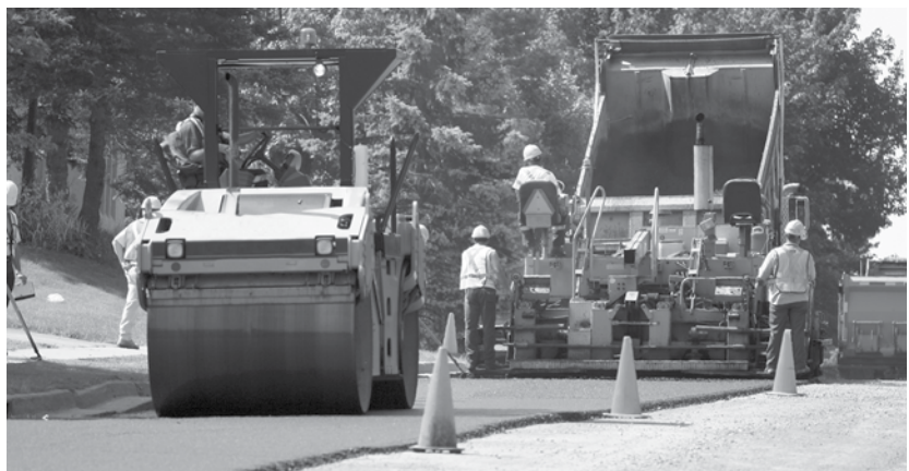
GPS technology can be used in a range of highway construction practices, including paving.
