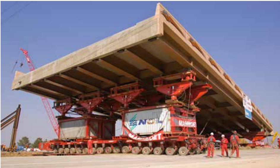
Today's innovative bridge technologies also include prefabricated bridge elements and systems. Here, the prefabricated superstructure of the 4500 South bridge in Salt Lake City, UT, is installed using a self propelled modular transporter.
