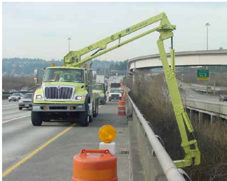
When conducting inspections, some bridge elements can only be reached using specialized equipment.
