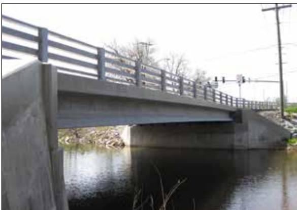
Ultra-high performance concrete (UHPC) is among the technologies promoted by FHWA’s Innovative Bridge Research and Deployment program. Structures that have used UHPC across the country include the Route 31 bridge in Lyons, NY.
