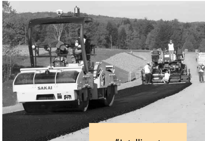
An intelligent compaction (IC) roller is used to place a hot-mix asphalt lift on U.S. 219 in Springville, NY.
