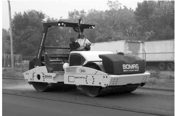
A thin lift of hot-mix asphalt is compacted with an IC roller on U.S. 52 in West Lafayette, IN.
