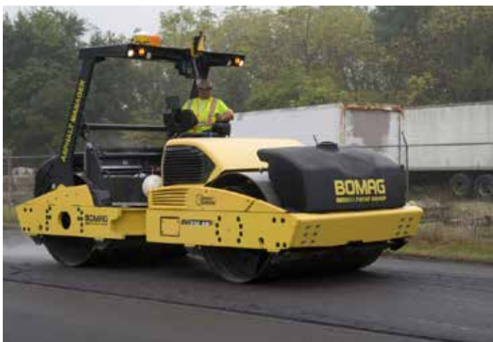
A thin lift of hot-mix asphalt is compacted with an intelligent compaction roller on U.S. 52 in West Lafayette, IN.
