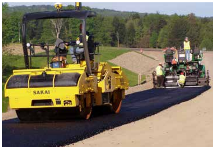
An intelligent compaction roller is used to place a hot-mix asphalt lift on U.S. 219 in Springville, NY.
