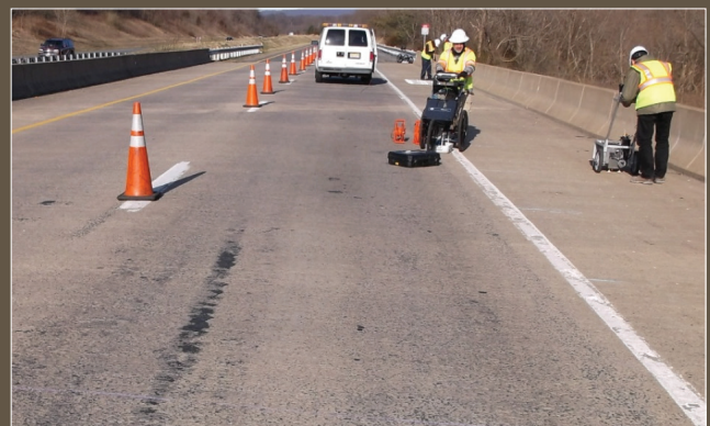
Figure 6. NDE survey on Virginia steel multigirder cluster bridge, Rt. 7 over South Fork of the Catoctin Creek.
