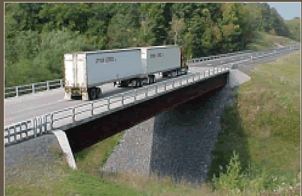
Figure 11. A double tractor trailer on a bridge. Source: Bala Sivakumar, HNTB Corporation.
