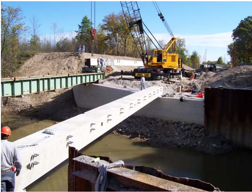
Geosynthetic reinforced soil (GRS) bridge system, Defiance County, Ohio.
