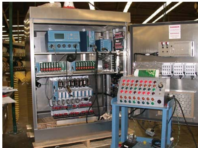
Traffic control signal box.
