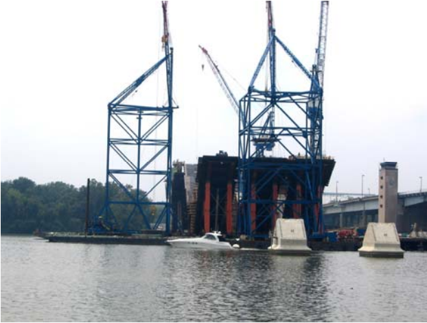
Construction of the Woodrow Wilson Bridge, outside of Washington, DC.
