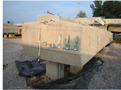
An instrumented concrete pile and cap collects strain and acceleration data.
