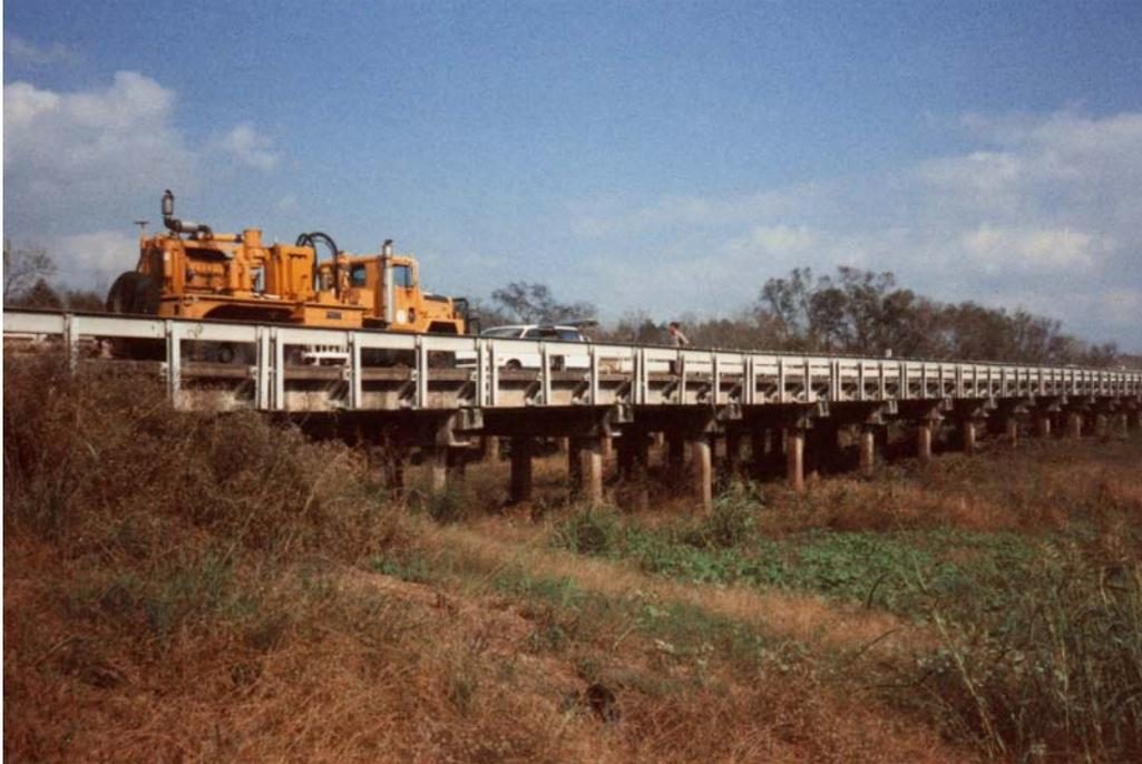
Figure 3. Photo. Relief structure 4 of the Trinity River Relief Bridge with the Vibroseis truck over bent 2.
