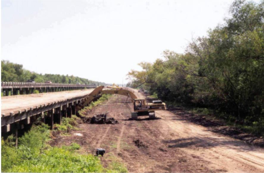
Figure 23. Photo. Backhoe excavation at bent 12, Trinity River Relief Bridge.
