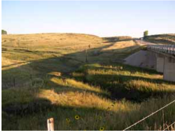
Figure 68. North Rush Creek, Great Plains—upstream of bridge.
