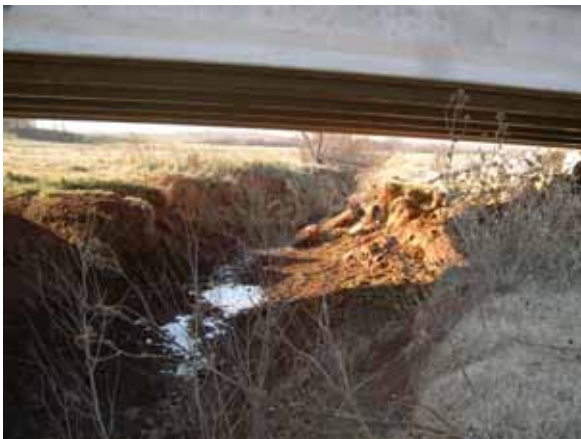
Figure 84. Beaver Creek, Central Plains— facing upstream under bridge.
