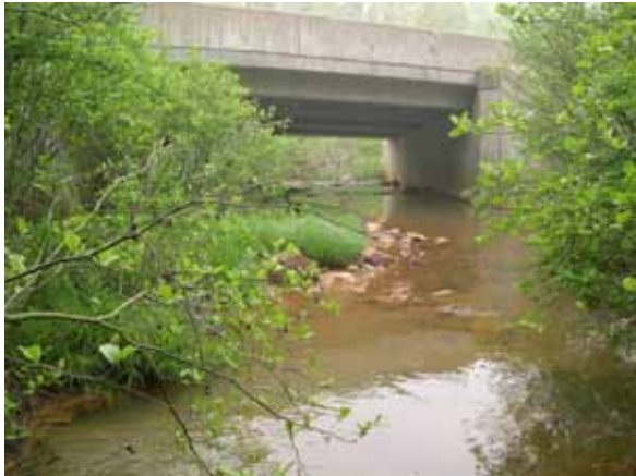
Figure 187. Unnamed creek (N 48), Appalachian Plateau— looking downstream at bridge.
