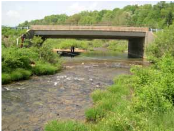
Figure 199. Sandy Creek, Appalachian Plateau— looking downstream at bridge.
