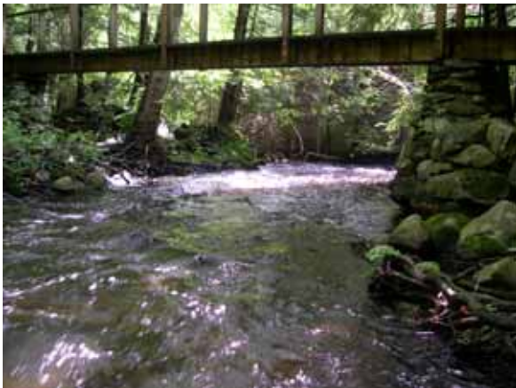
Figure 171. West Branch Saugatuck River, New England— looking downstream at bridge (bridge in foreground is the pedestrian bridge).
