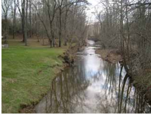
Figure 8. Failing banks in the Interior Lowlands.
