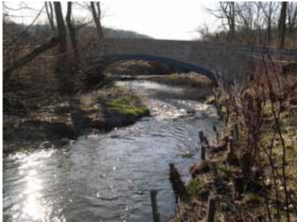
Figure 211. Indian Run, Piedmont— looking downstream at bridge.
