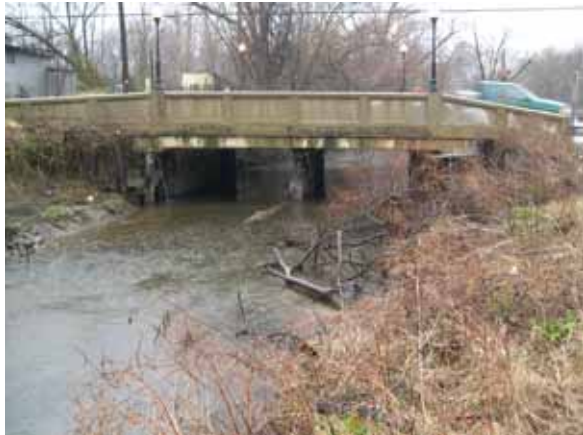
Figure 143. Mill Stream Branch, Atlantic Coastal Plain—looking downstream at bridge.
