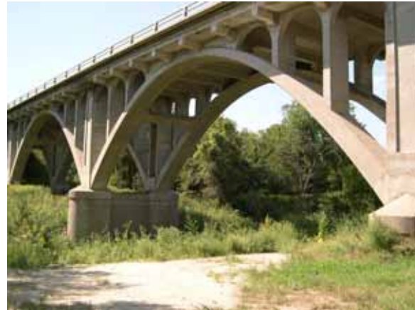
Figure 73. Saline River, Great Plains—looking downstream at bridge.
