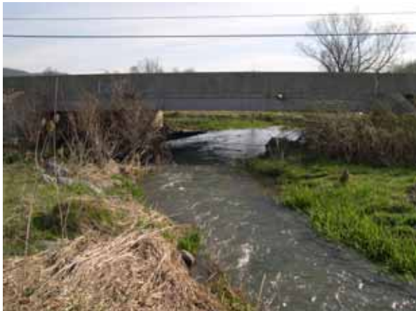
Figure 231. Buffalo Run, Valley and Ridge—looking downstream at bridge.
