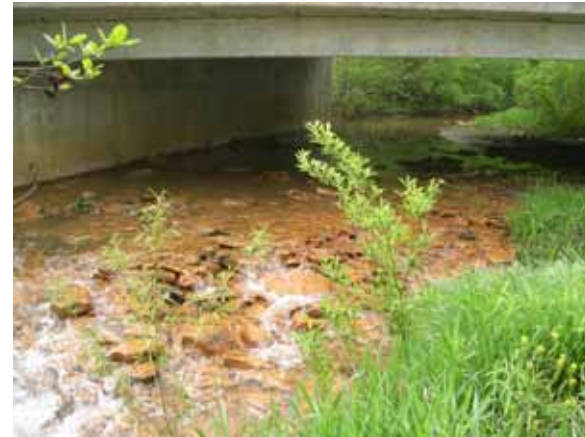
Figure 188. Unnamed creek (N 48), Appalachian Plateau— looking upstream through bridge.
