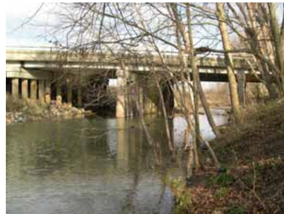
Figure 128. Unnamed creek (N 24), Atlantic Coastal Plain—looking downstream at bridge.
