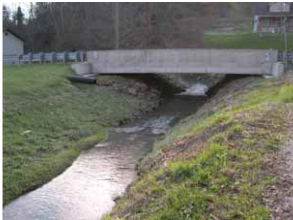
Figure 179. McKnownn Creek, Appalachian Plateau— looking downstream at bridge.
