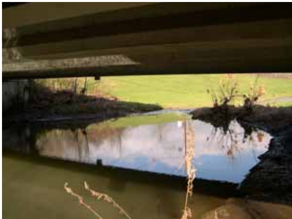
Figure 103. Unnamed creek (N 28), Interior Low Plateau— downstream under bridge.
