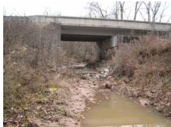
Figure 124. Unnamed creek (N 23), Atlantic Coastal Plain— looking upstream at bridge.
