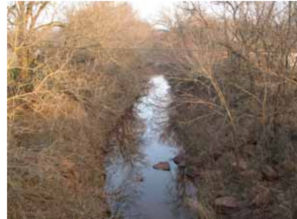
Figure 87. Brush Creek, Central Plains— downstream from bridge.
