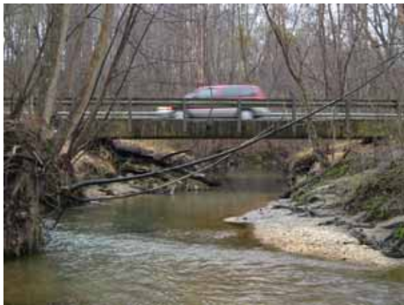
Figure 139. Stocketts Run, Atlantic Coastal Plain— looking downstream at bridge.
