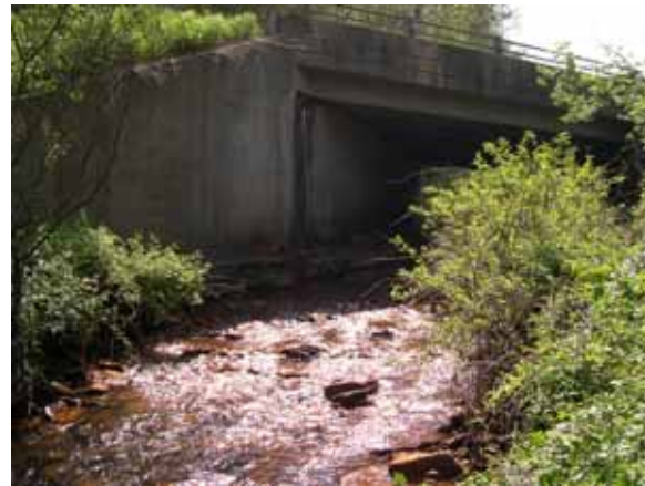
Figure 192. Reids Run, Appalachian Plateau— looking upstream at bridge.
