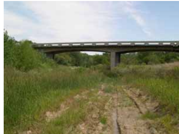
Figure 75. South Fork Solomon River, Great Plains— looking downstream at bridge, photo 2.
