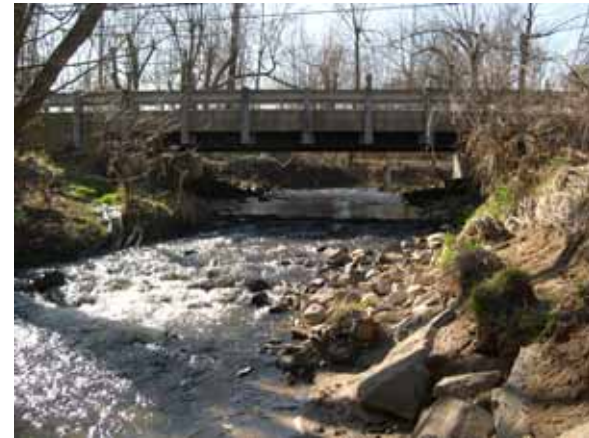
Figure 156. Hammond Branch, Atlantic Coastal Plain—looking upstream at bridge.
