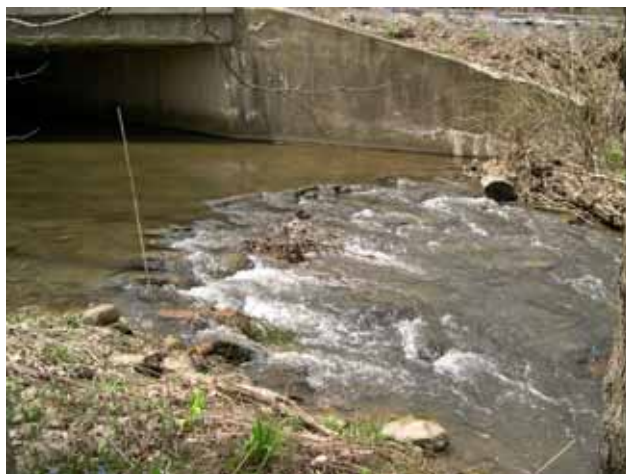
Figure 17. Cross vane downstream of bridge over Potter Run, PA.
