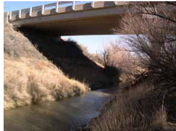
Figure 60. Rio San Jose, Trans Pecos— looking downstream at bridge.
