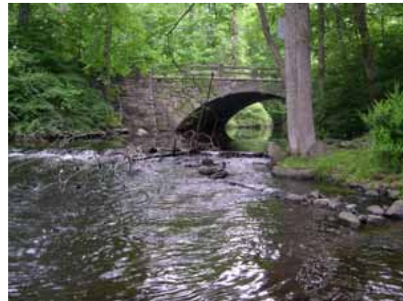
Figure 176. Mianus River, New England— looking upstream at bridge.
