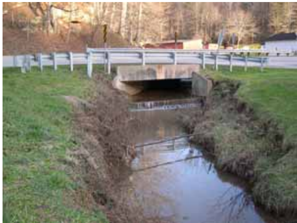
Figure 183. Wolf Run, Appalachian Plateau—looking upstream at bridge.
