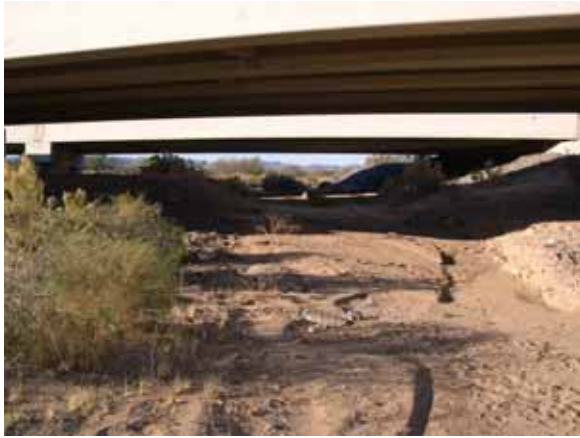
Figure 49. Sacramento Wash, Basin and Range— upstream under bridge.
