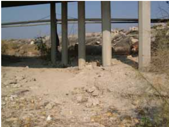
Figure 31. Buena Vista Creek, Pacific Coastal— downstream under bridge.
