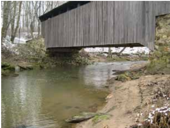
Figure 223. Little Elk Creek, Piedmont— looking upstream at bridge.
