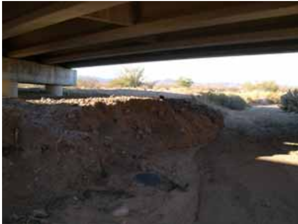
Figure 51. Sacramento Wash, Basin and Range— downstream under bridge.
