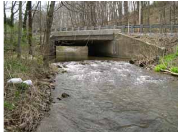
Figure 240. Potter Run, Valley and Ridge— looking upstream at bridge.
