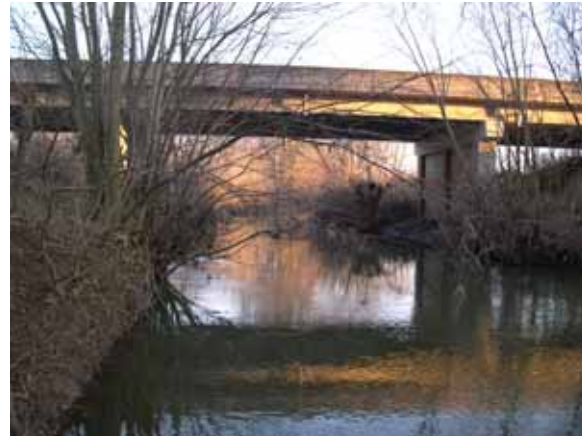
Figure 108. South Fork, Interior Low Plateau— looking downstream at bridge.
