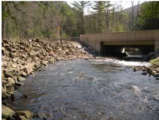
Figure 16. Riprap stabilization wall along Roaring Run, PA.
