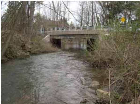
Figure 239. Potter Run, Valley and Ridge— looking downstream at bridge.
