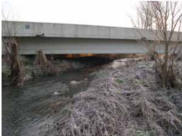
Figure 95. East Fork, Interior Low Plateau— looking upstream at bridge.
