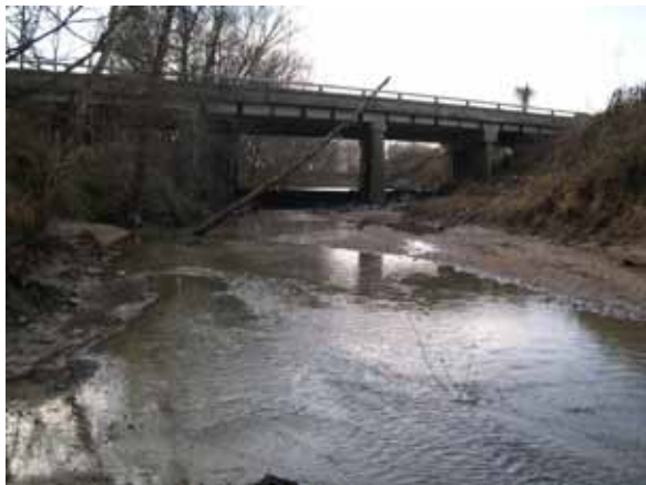
Figure 127. Unnamed creek (N 24), Atlantic Coastal Plain—looking upstream at bridge.
