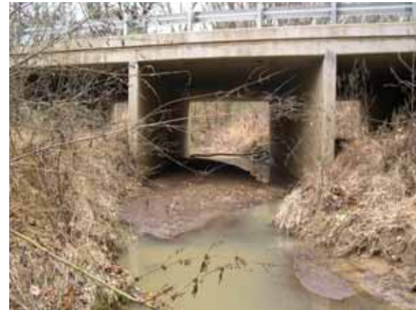
Figure 120. Little Cypress Creek, Atlantic Coastal Plain— looking upstream at bridge.
