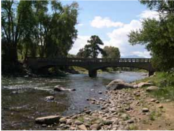
Figure 61. Arkansas River, Rocky Mountains— looking downstream at bridge.
