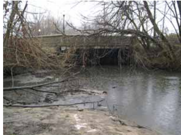
Figure 144. Mill Stream Branch, Atlantic Coastal Plain—looking upstream at bridge.
