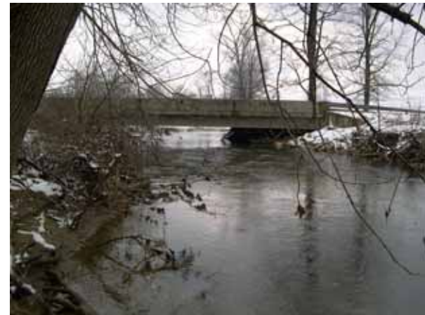
Figure 228. Big Beaver Creek, Piedmont—looking upstream at bridge.
