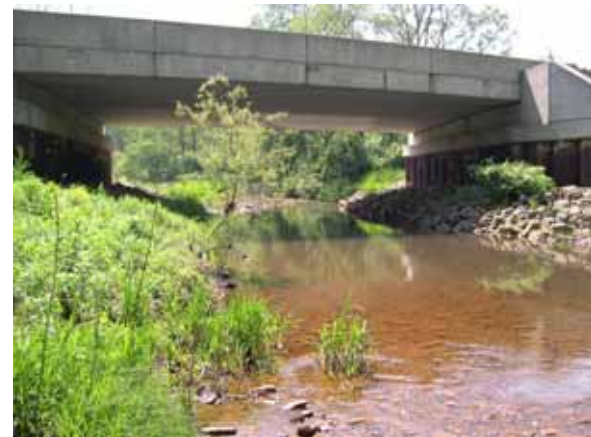
Figure 196. Piney Creek, Appalachian Plateau— looking upstream at bridge.
