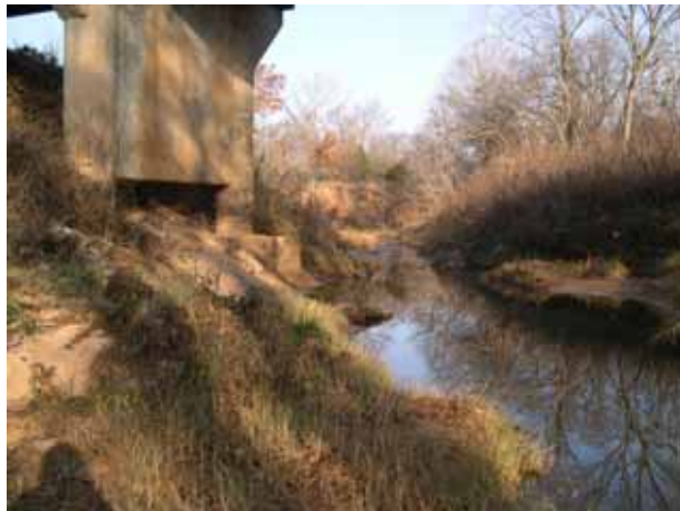
Figure 7. Failing banks in the Central Lowlands.
