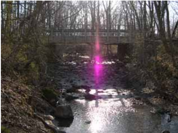
Figure 219. Atherton Tributary, Piedmont—looking upstream at bridge.
