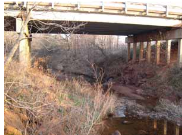
Figure 88. Brush Creek, Central Plains— downstream under bridge.
