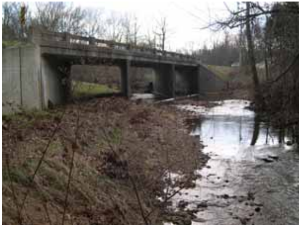
Figure 99. Honey Run, Interior Low Plateau— looking upstream at bridge.
