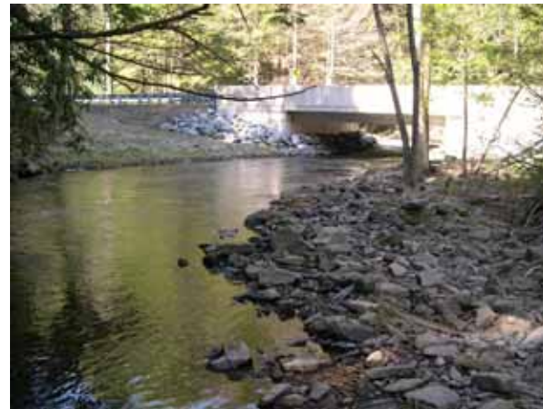
Figure 236. Roaring Run, Valley and Ridge—looking upstream at bridge.
