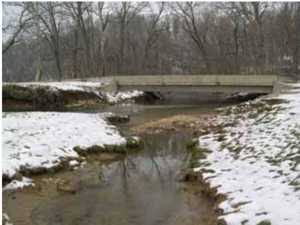
Figure 227. Big Beaver Creek, Piedmont—looking downstream at bridge.
