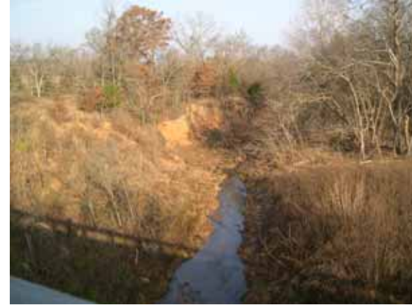
Figure 90. Unnamed creek (N 19), Central Plains— upstream from bridge.
