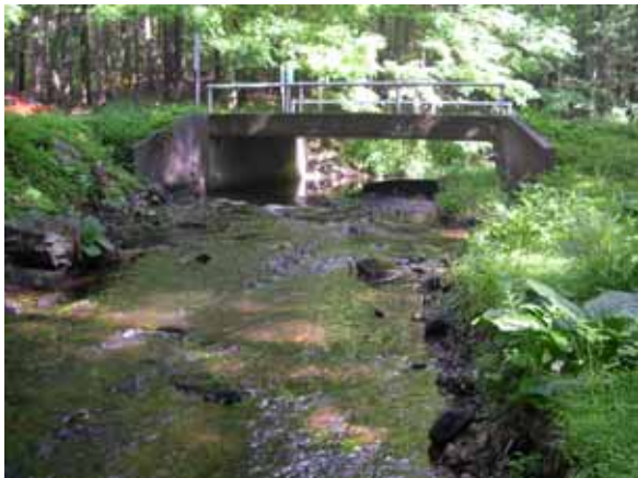
Figure 163. Mill River, New England— looking upstream at bridge.
