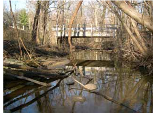
Figure 220. Atherton Tributary, Piedmont—looking downstream at bridge.
