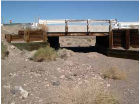
Figure 47. Rt. 66 Wash, Basin and Range—looking downstream at bridge.
