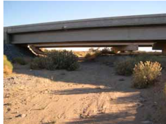
Figure 52. Sacramento Wash, Basin and Range— looking downstream at bridge.
