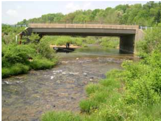
Figure 14. Meander migration affecting right abutment, Hammond Branch, MD.
