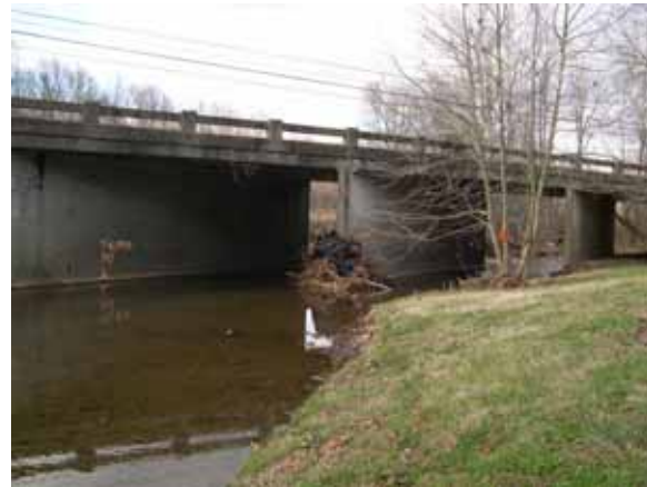
Figure 100. Honey Run, Interior Low Plateau— looking downstream at bridge.
