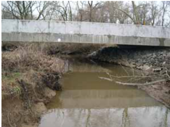
Figure 151. Morgan Creek, Atlantic Coastal Plain— looking upstream at bridge.
