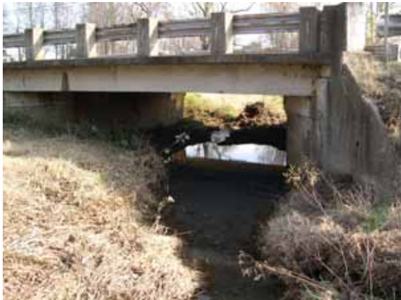
Figure 115. Unnamed creek (N 21), Ozark-Ouachita Highlands— looking downstream at bridge.
