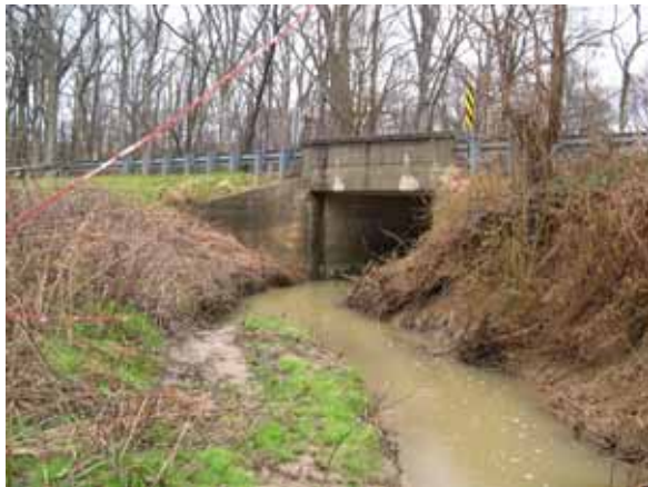
Figure 147. Kent County Tributary, Atlantic Coastal Plain—looking downstream at bridge.
