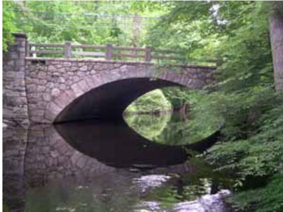
Figure 175. Mianus River, New England— looking downstream at bridge.
