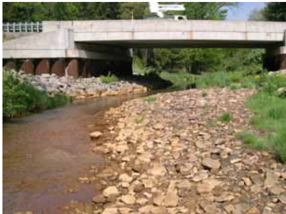
Figure 195. Piney Creek, Appalachian Plateau— looking downstream at bridge.
