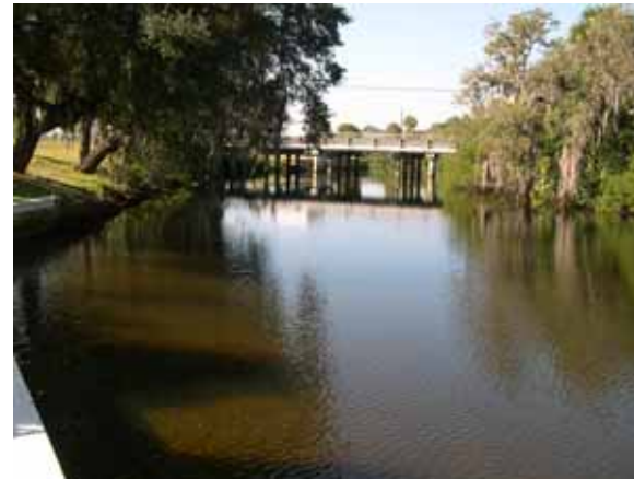
Figure 134. Alligator Creek, Atlantic Coastal Plain— looking downstream at bridge.
