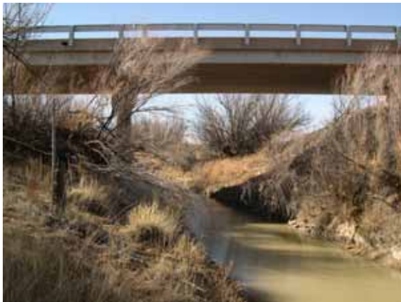
Figure 59. Rio San Jose, Trans Pecos— looking upstream at bridge.
