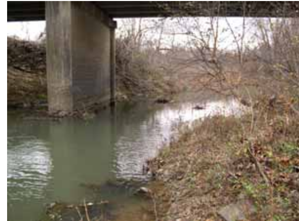
Figure 112. Little Skin Creek, Ozark-Ouachita Highlands— looking downstream at bridge (right).
