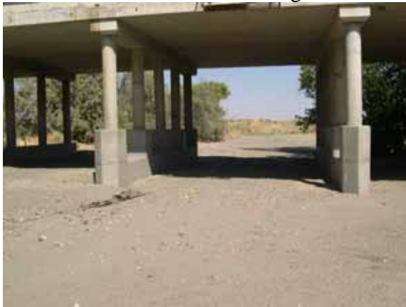
Figure 35. Jacalitos Creek, Pacific Coastal— looking downstream at bridge.
