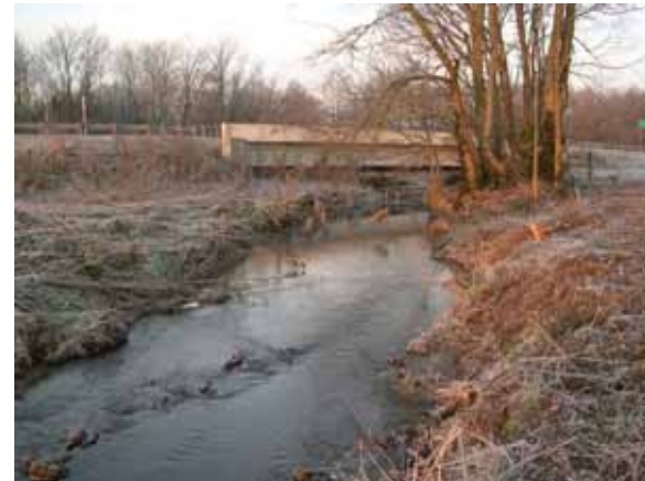
Figure 96. East Fork, Interior Low Plateau— looking downstream at bridge.
