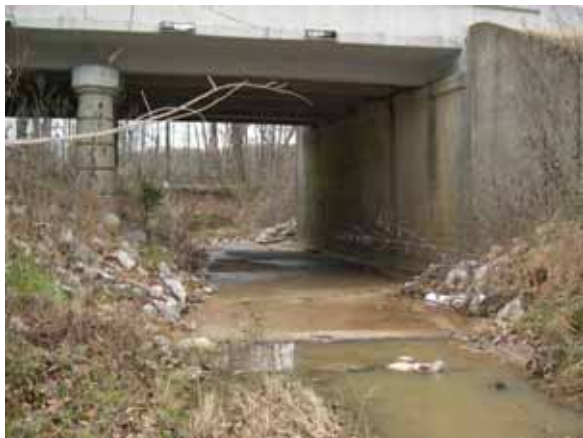
Figure 123. Unnamed creek (N 23), Atlantic Coastal Plain— looking downstream at bridge.
