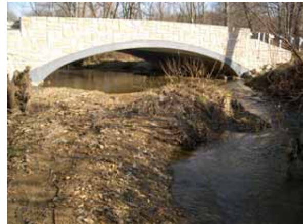
Figure 212. Indian Run, Piedmont— looking upstream at bridge.
