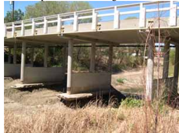
Figure 40. Murietta Creek, Pacific Coastal— looking upstream at bridge.
