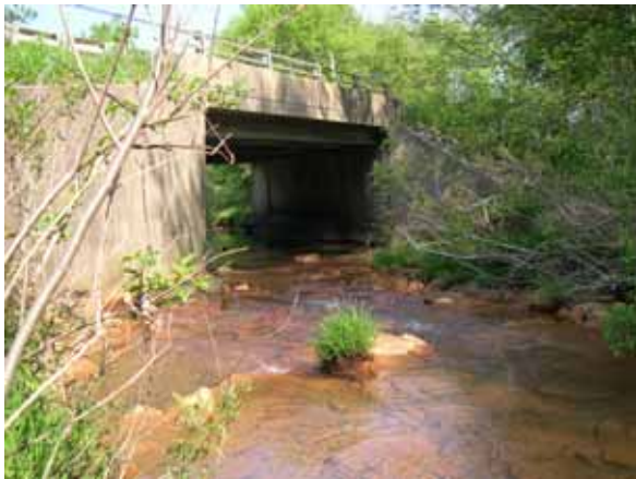
Figure 191. Reids Run, Appalachian Plateau— looking downstream at bridge.
