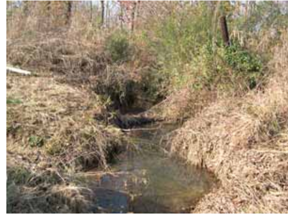
Figure 114. Unnamed creek (N 21), Ozark-Ouachita Highlands— upstream from bridge.
