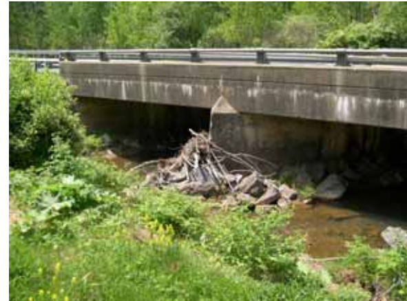
Figure 204. Trout Run, Appalachian Plateau— upstream face of bridge.
