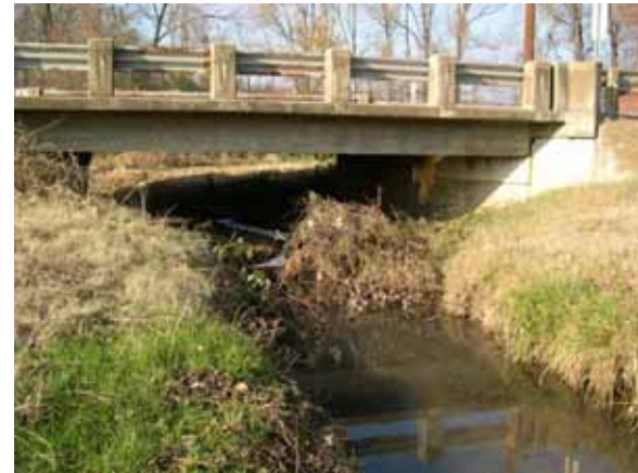
Figure 116. Unnamed creek (N 21), Ozark-Ouachita Highlands— looking upstream at bridge.
