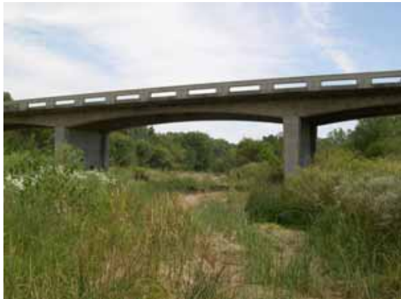
Figure 74. South Fork Solomon River, Great Plains— looking downstream at bridge, photo 1.
