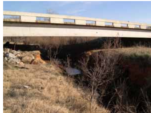
Figure 85. Beaver Creek, Central Plains— facing downstream under bridge.
