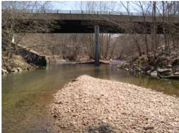
Figure 215. Middle Patuxent River, Piedmont—looking downstream at bridge.
