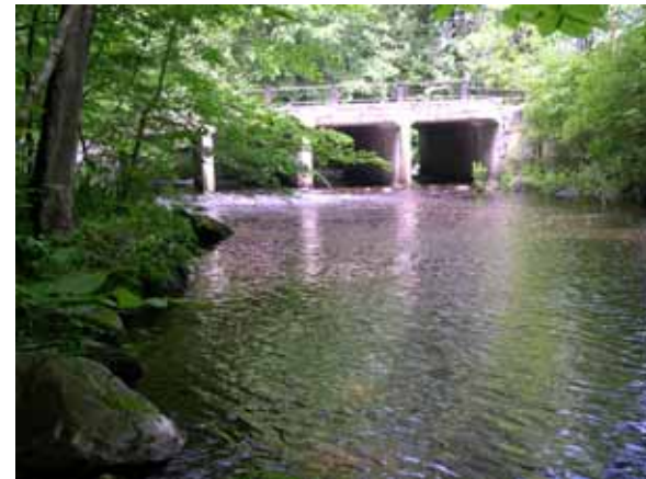
Figure 172. West Branch Saugatuck River, New England— looking upstream at bridge.
