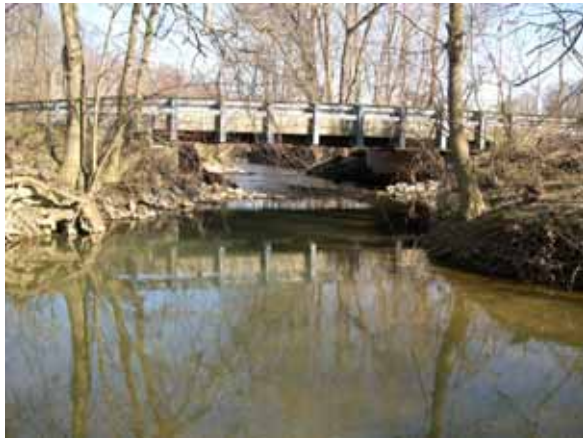
Figure 155. Hammond Branch, Atlantic Coastal Plain—looking downstream at bridge.
