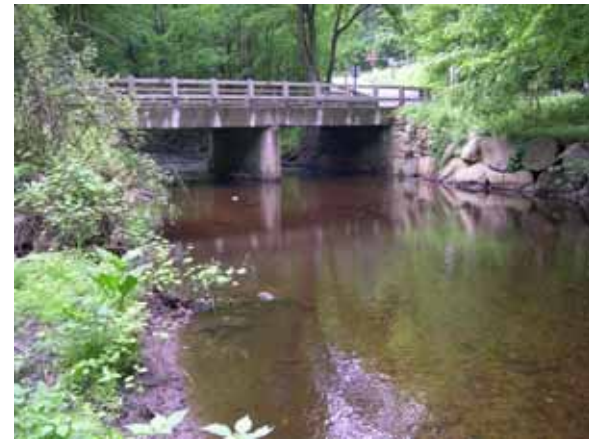
Figure 168. Aspetuck River, New England— looking downstream at bridge.
