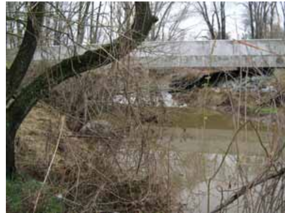
Figure 152. Morgan Creek, Atlantic Coastal Plain— looking downstream at bridge.
