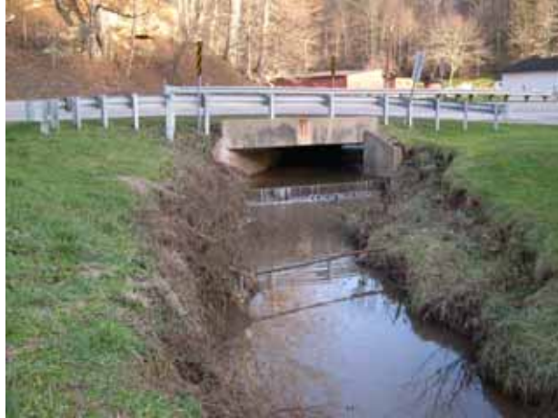
Figure 15. Single-span bridge over unstable channel.
