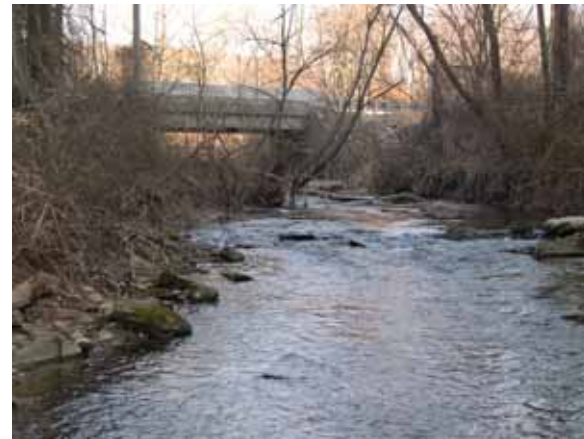
Figure 208. Blackrock Run, Piedmont— looking upstream at bridge.
