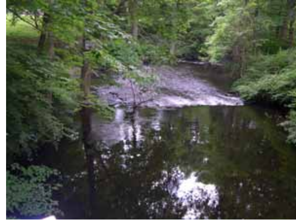
Figure 174. Mianus River, New England— downstream from bridge. Note weir.
