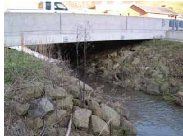
Figure 180. McKnownn Creek, Appalachian Plateau— looking upstream at bridge.
