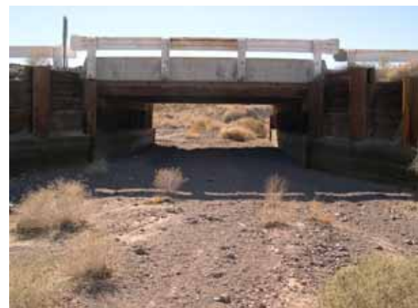
Figure 48. Rt. 66 Wash, Basin and Range—looking upstream at bridge.
