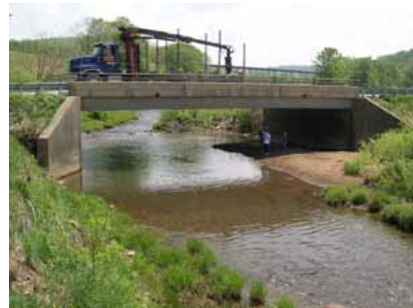
Figure 200. Sandy Creek, Appalachian Plateau— looking upstream at bridge.
