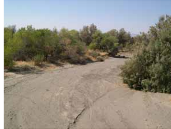
Figure 34. Jacalitos Creek, Pacific Coastal— upstream from bridge.
