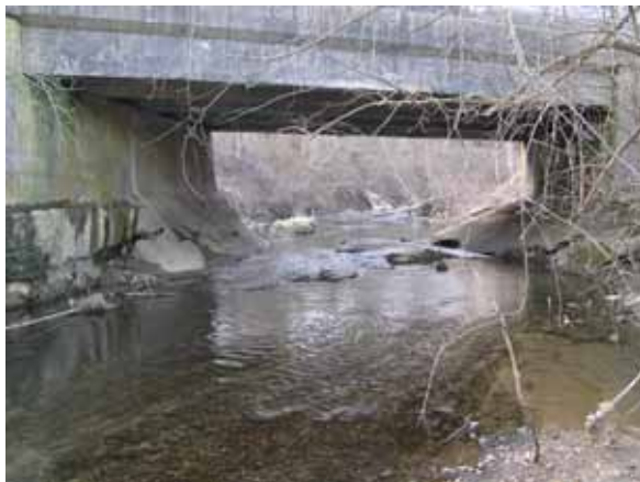
Figure 207. Blackrock Run, Piedmont— looking downstream at bridge.
