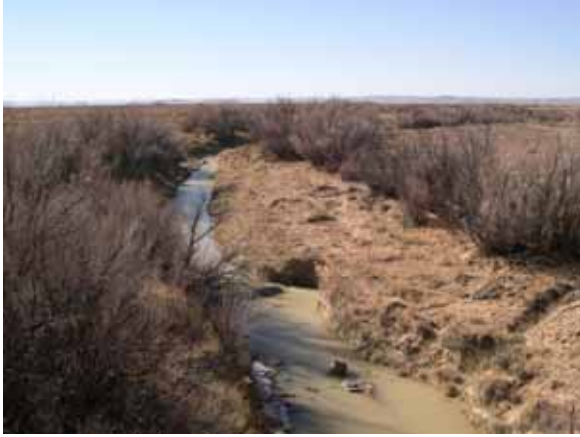
Figure 57. Rio San Jose, Trans Pecos— upstream from bridge.
