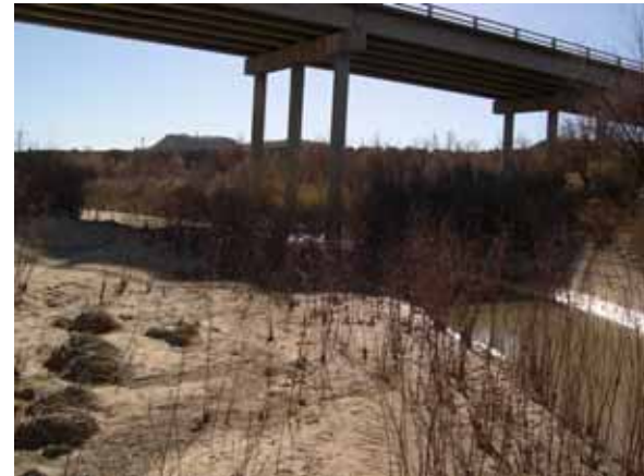
Figure 56. Rio Puerco, Trans Pecos— looking downstream at bridge.
