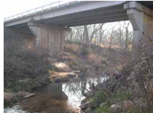
Figure 92. Unnamed creek (N 19), Central Plains— downstream under bridge.
