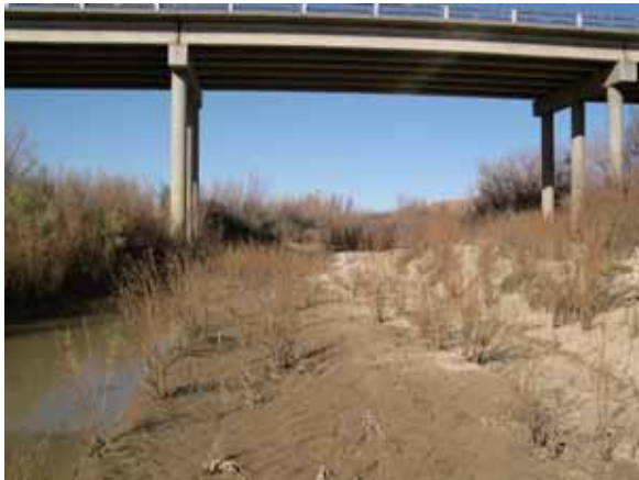
Figure 55. Rio Puerco, Trans Pecos— looking upstream at bridge.
