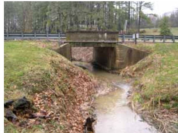
Figure 148. Kent County Tributary, Atlantic Coastal Plain—looking upstream at bridge.
