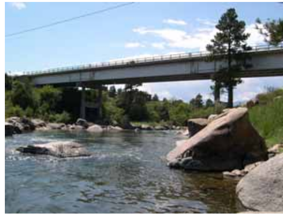
Figure 64. Arkansas River, Rocky Mountains— bridge #2 downstream from other bridge.
