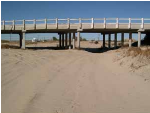
Figure 43. Mojave River, Basin and Range—looking downstream at bridge.
