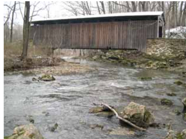
Figure 224. Little Elk Creek, Piedmont— looking downstream at bridge.
