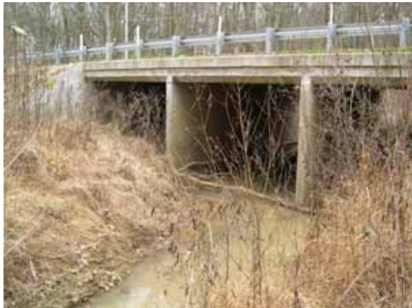
Figure 119. Little Cypress Creek, Atlantic Coastal Plain— looking downstream at bridge.
