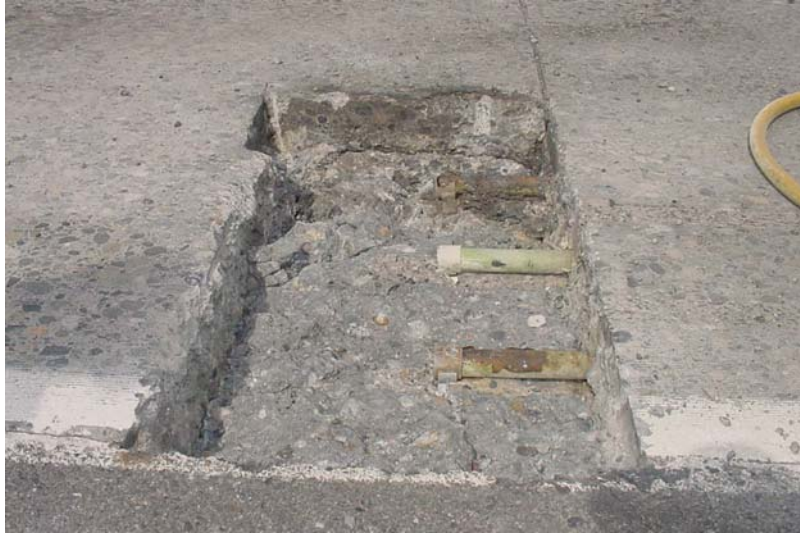
Figure 1. Photo. Exposed failures with rusted dowel bars (Washington State Department of Transportation Pavement Guide). (4)
