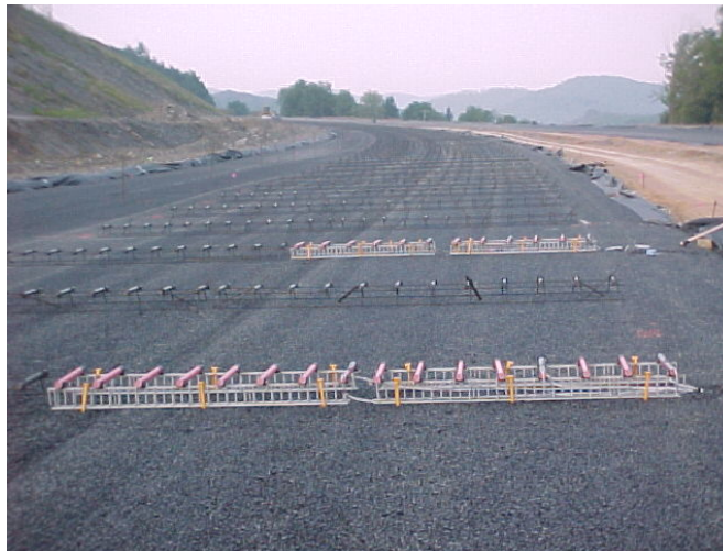
Figure 55. Photo. Dowel installation at location 1 of corridor H, Route 250, Elkins, WV.
