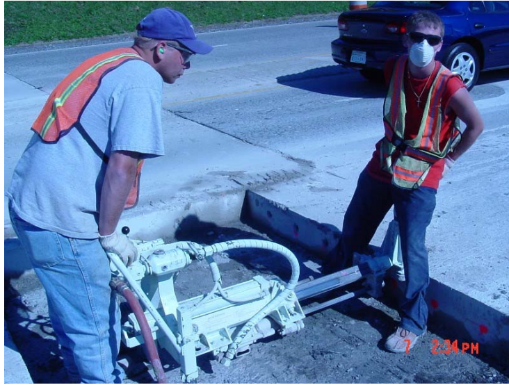
Figure 88. Photo. Drilling holes for inserting dowels.
