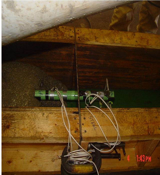
Figure 10. Photo. Dowel being covered by concrete.
