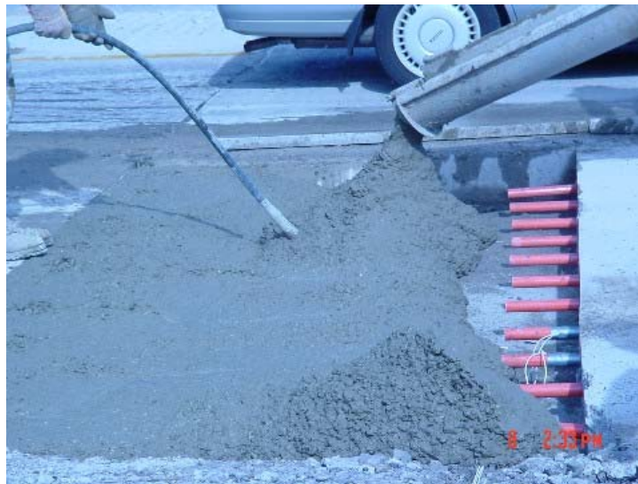
Figure 91. Photo. Concrete placement and vibration.
