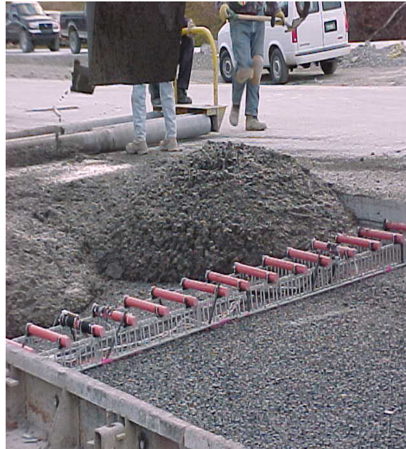
Figure 62. Photo. Paving operation in progress.
