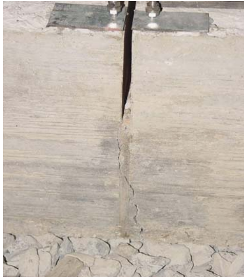
Figure 18. Photo. Typical crack observed in slabs number 1, 4, and 5 (table 7).
