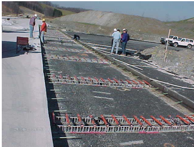
Figure 57. Photo. FRP dowel bars at location 2 of corridor H, Route 219, Elkins, WV.
