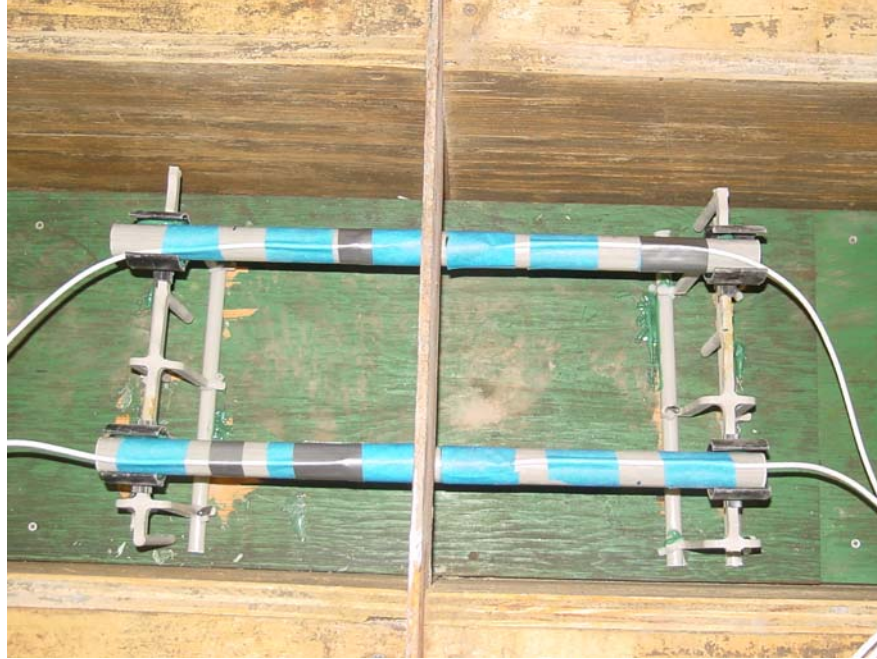
Figure 8. Photo. Instrumented dowels and steel plate positioned in the wood formwork.
