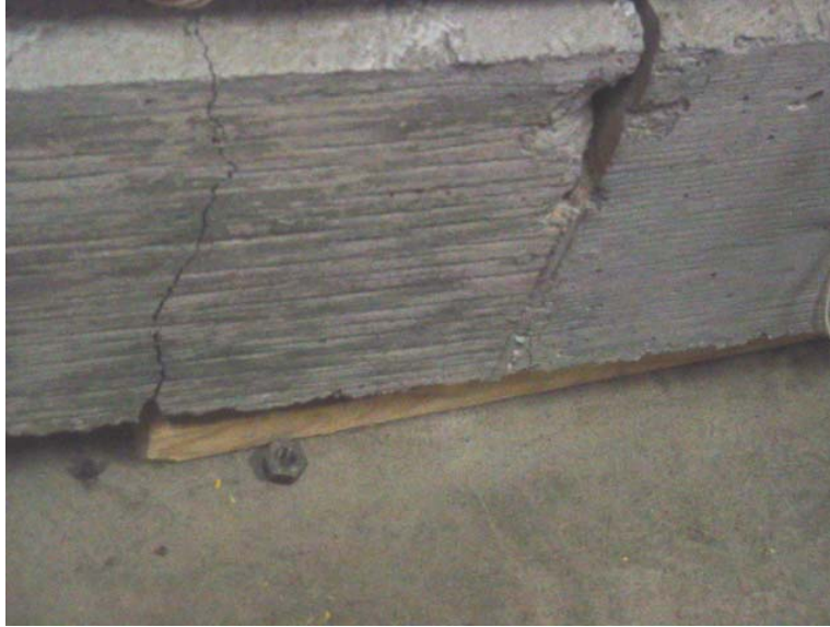
Figure 20. Photo. Typical crack observed in slab number 3 (table 7).
