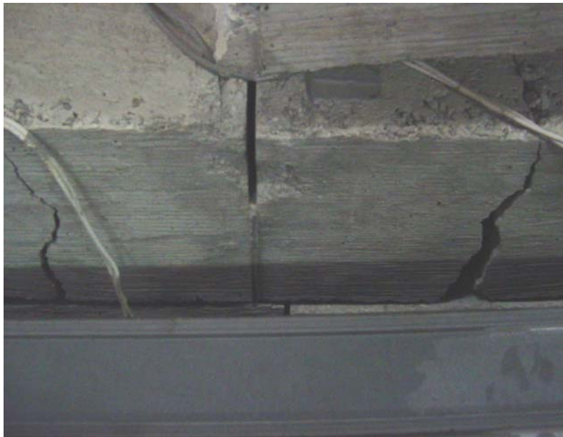
Figure 19. Photo. Crack observed in slab number 2 (table 7).
