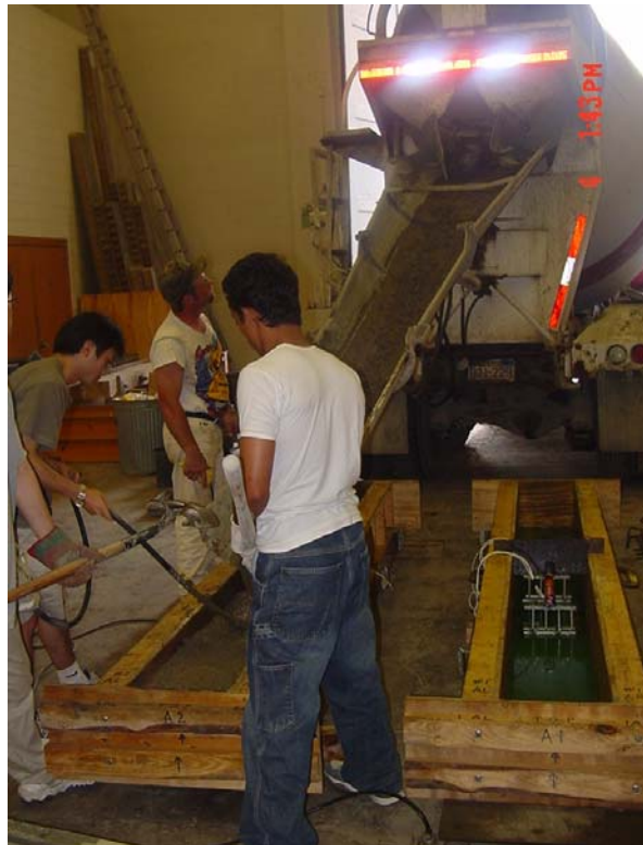
Figure 9. Photo. Placing concrete into the formwork.
