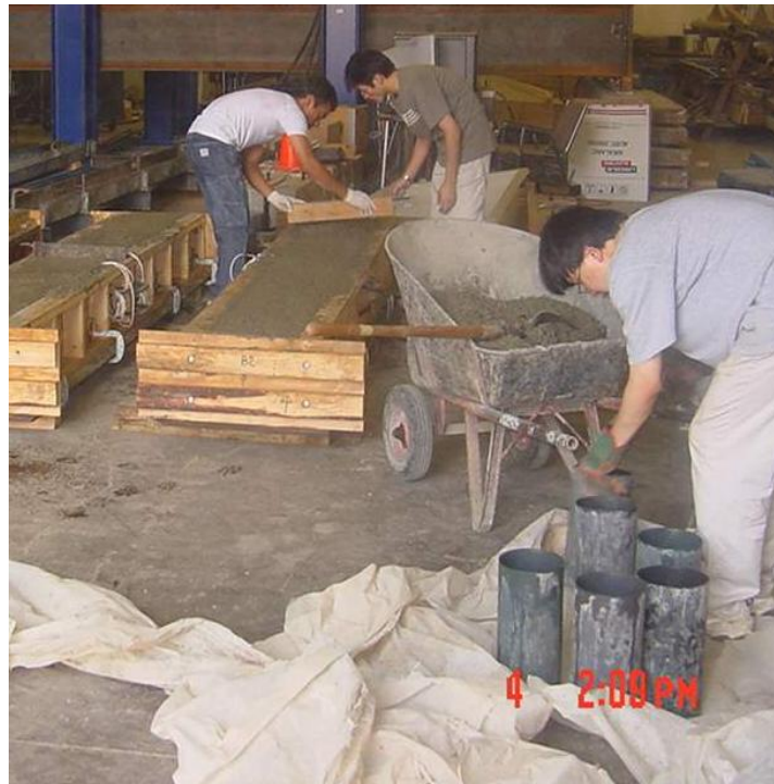
Figure 11. Photo. Casting concrete cylinders.
