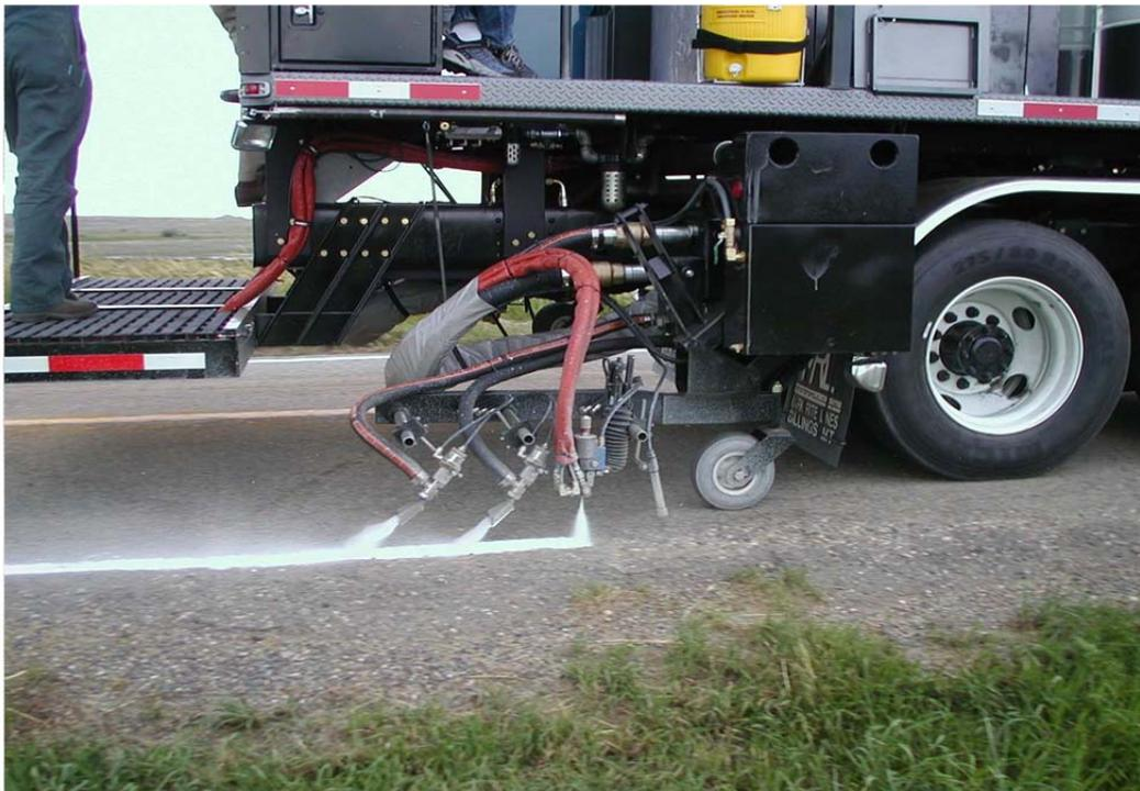
**Figure 11. Photo. Application of glass beads to long line markings.**
