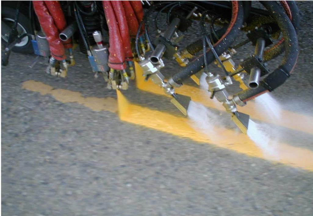
**Figure 12. Photo. Close-up of glass bead application to long lines.**
