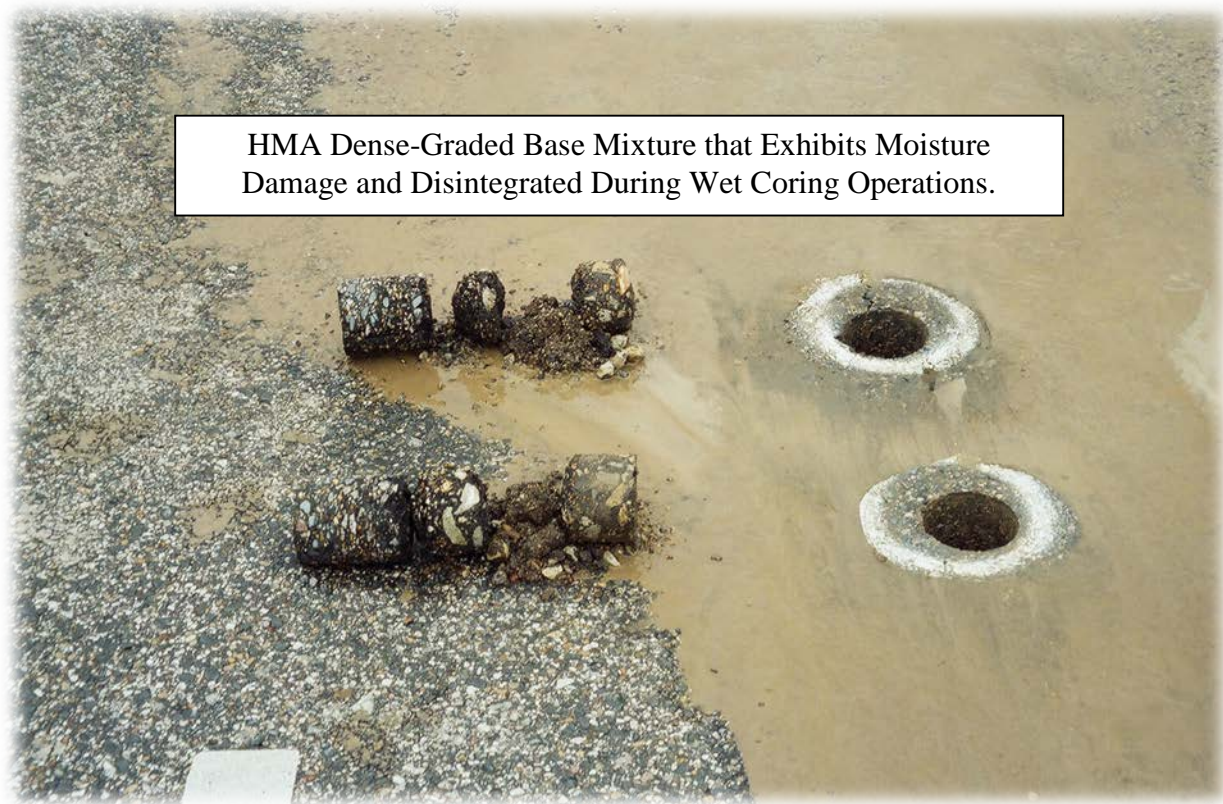
Figure 34. Photo. Cores recovered where moisture damage occurred, decreasing the in-place modulus of the layer/mixture (Texas SPS-5 project).
