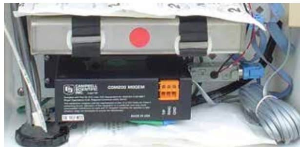
FIGURE C.2. Modem attached to Datalogger for transmitting data via landline to the respective LTPP regional support contractor's office computer.
