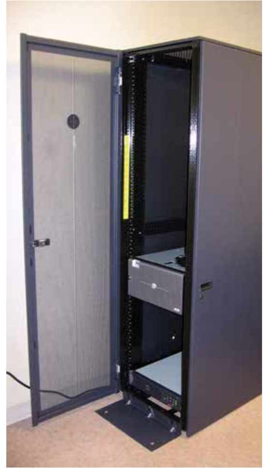
FIGURE 8.9. Dell™ PowerEdge™ 2900III installed in May 2009 at FHWA's Turner-Fairbank Highway Research Center to serve as the secure central repository for LTPP electronic data into the future. The server contains 8 TB disk storage, dual quad core Xeon® 3 GHz processors, 32 GB RAM, and the Windows® Server 2008 64-bit operating system.
