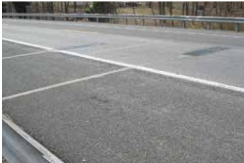
FIGURE 7.10. Staggered bending plate WIM sensors installed in concrete pavement.
