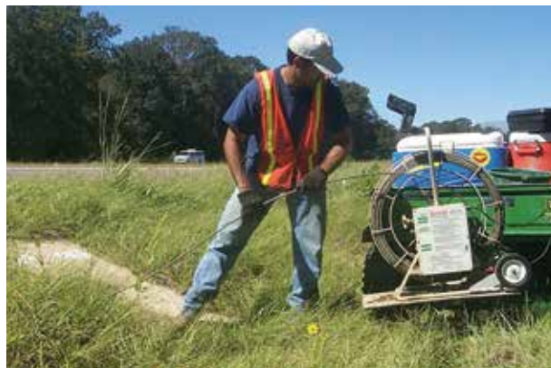
FIGURE 6.15. Edge drain inspection using videography.
