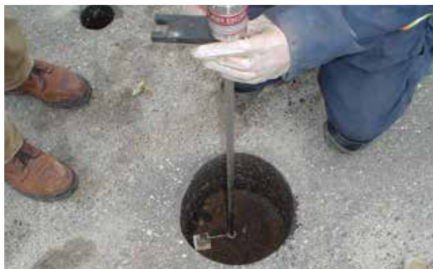
FIGURE 7.13. LTPP regional support contractor staff use the dynamic core penetrometer to determine the strength and density of the subgrade at the SPS-5 site in Minnesota.
