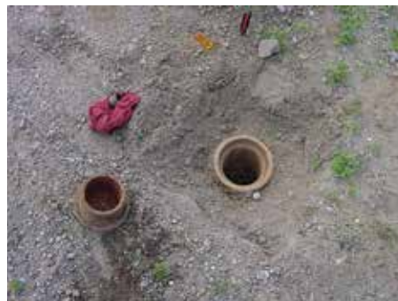
FIGURE 7.2. A piezometer monitoring well and cap, used to determine ground water levels.
