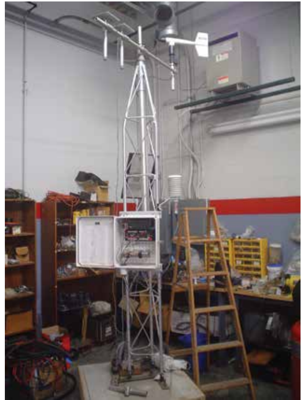
FIGURE 6.3. Prototype automated weather station used by the LTPP regional support contractors for in-house training of staff and to calibrate equipment components.
