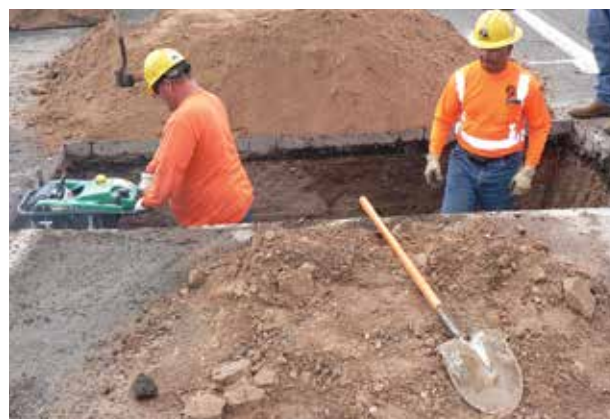
FIGURE 7.14. Workers prepare a trench for forensic investigation of an SPS-5 test site in Arizona.
