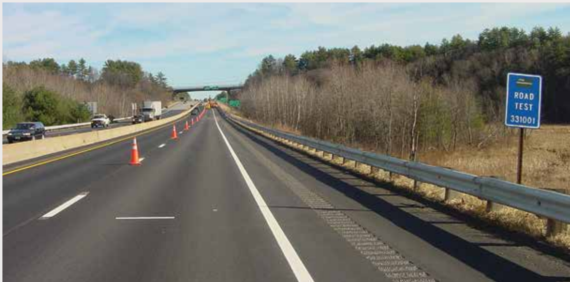
LTPP test site 331001 in New Hampshire (GPS-1: asphalt concrete on granular base). In the unique six-digit identifier, the first two digits indicate the State or Province where the test site is located.
