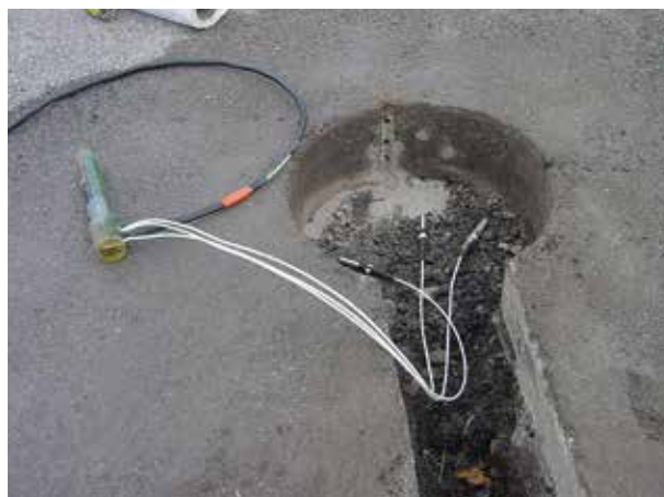
FIGURE C.6. "Piglet" style mini-probes installed to replace failed thermistor probes in Phase II of the Seasonal Monitoring Program.
