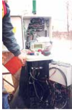
FIGURE 7.6. SMP Phase II seasonal monitoring equipment installation at the Lake Ontario State Parkway site on SR 947A in western New York.
