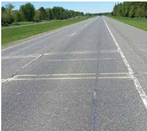
FIGURE 7.11. Installation of quartz piezoelectric WIM sensor spanning a full lane.
