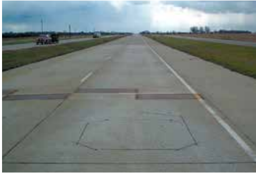
FIGURE 7.9. Load cell WIM installation.
