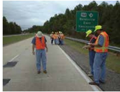
FIGURE 9.2. Distress raters evaluate a pavement surface in an LTPP accreditation workshop, where raters' proficiency is tested.
