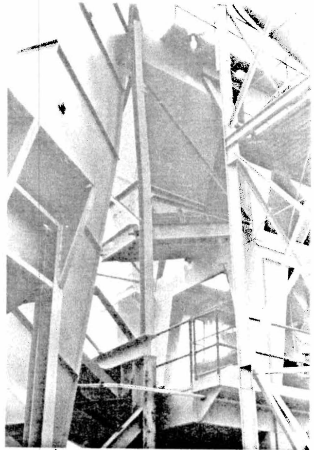
FIGURE 6 Surge Hopper and Drag-Out Belt
