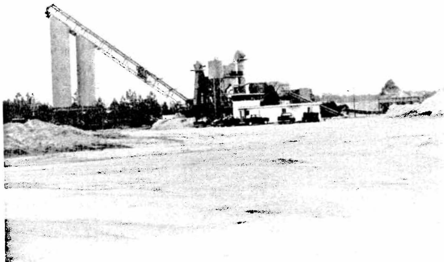
FIGURE 4 Batch Plant Used to Process Recycled Mixture
