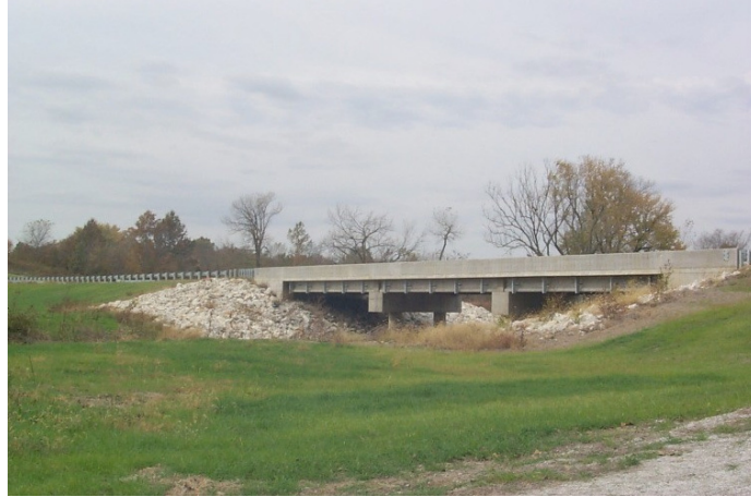
Figure 33. Side view of Bridge Number 6059.
