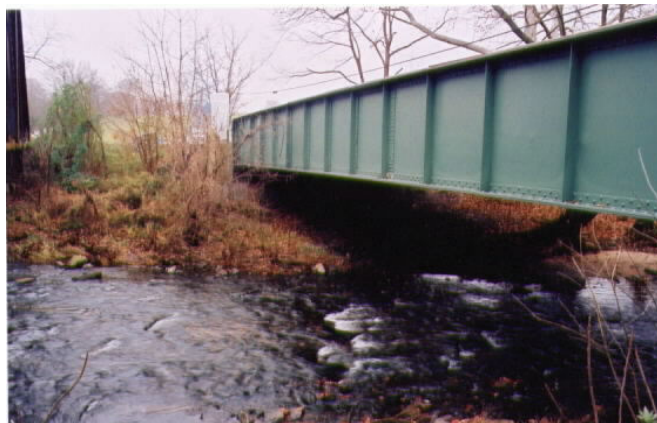
Figure 6. Side view of Bridge No. 1-119.
