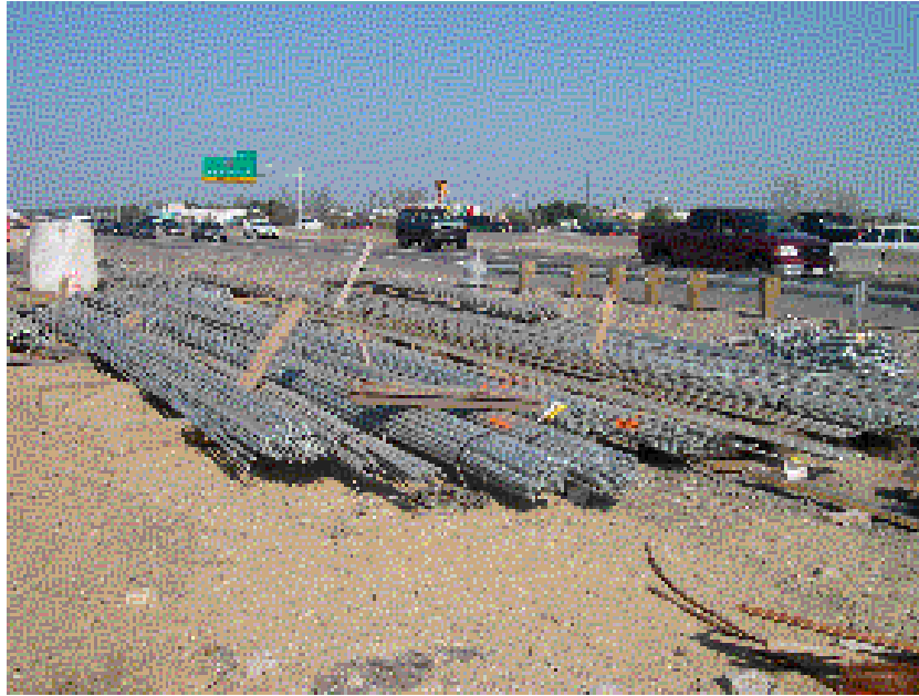
Figure 47. Bundled/wrapped bars at the Frontage Road job site.
