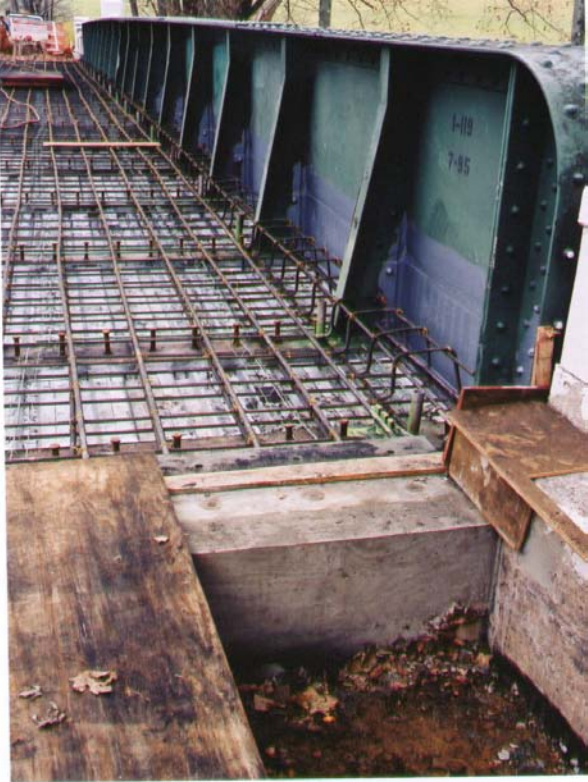
Figure 8. General view of in-place reinforcement, girders with studs, curb, and bulkhead.
