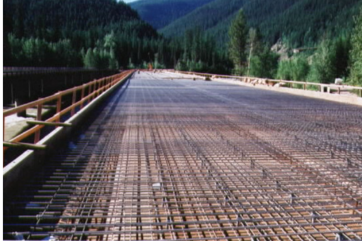
Figure 35. View of deck with stainless steel reinforcement placement in progress.
