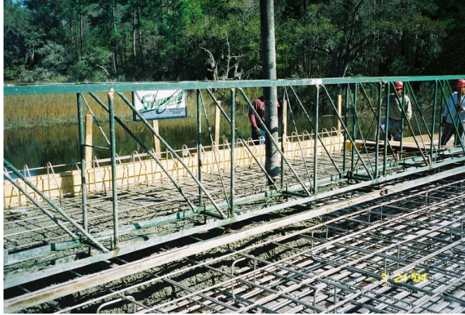
Figure 65. View of in-place clad stainless in span 3.
