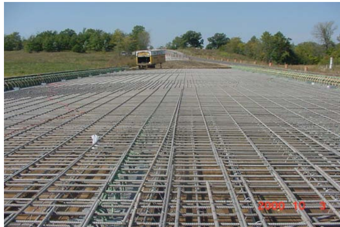
Figure 34. View of bridge deck with stainless steel in place.
