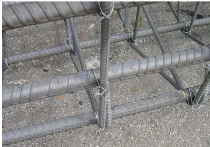
Figure 24. Closeup view of a portion of the 2201 ss reinforcing bars in the column cage prior to placement in pier number 11.
