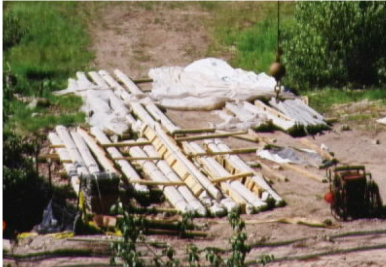
Figure 36. Photograph of bundled/wrapped bars at the job site.
