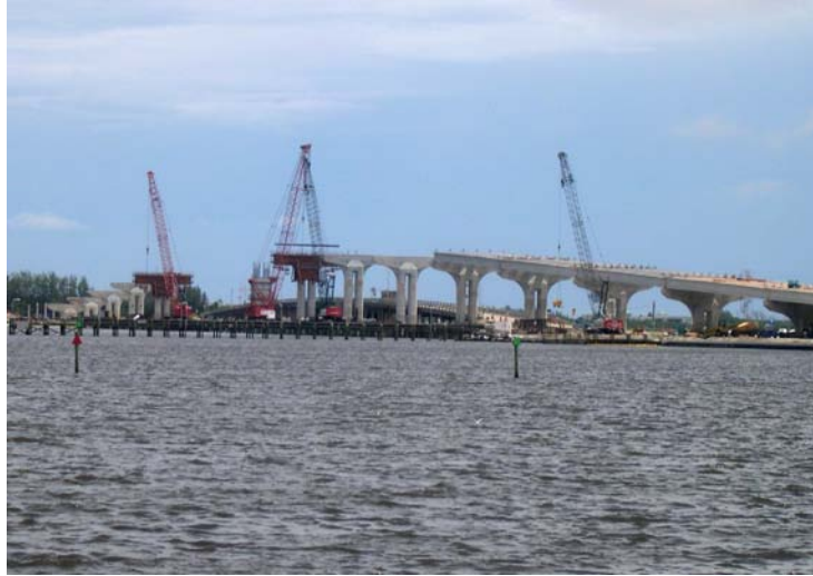
Figure 18. Perspective photograph of the Jensen Beach Causeway Bridge under construction.
