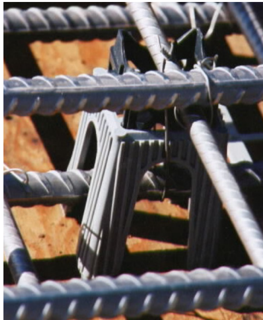
Figure 42. Closeup view of a plastic chair to which bars are tied.
