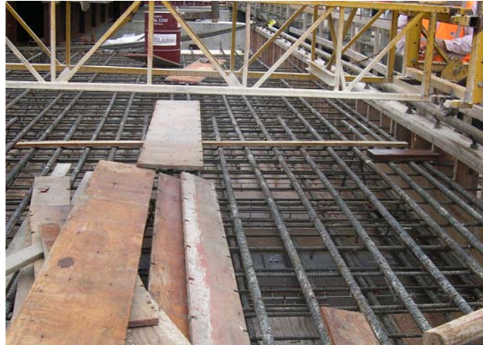
Figure 16. Second view of MMFX-II deck steel in place.
