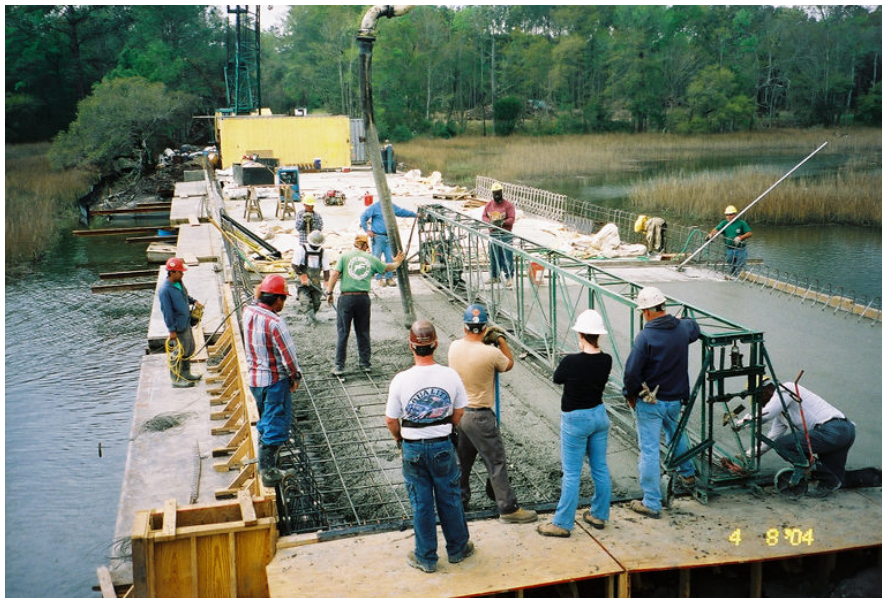
Figure 62. General view of the bridge under construction.
