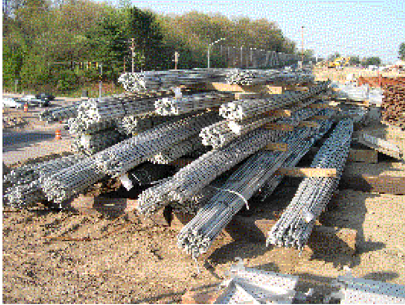
Figure 49. Stored galvanized bars at the Brown Avenue Bridge job site.
