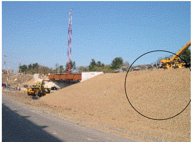
Figure 44. General view of the Brown Avenue Bridge under construction.
