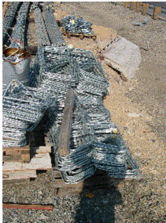
Figure 48. Fabricated galvanized bars at the Frontage Road Bridge job site.
