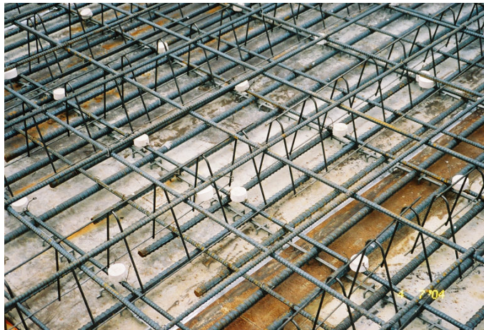
Figure 67. Closeup view of discrete galvanic anodes on in-place span 1 black bars.
