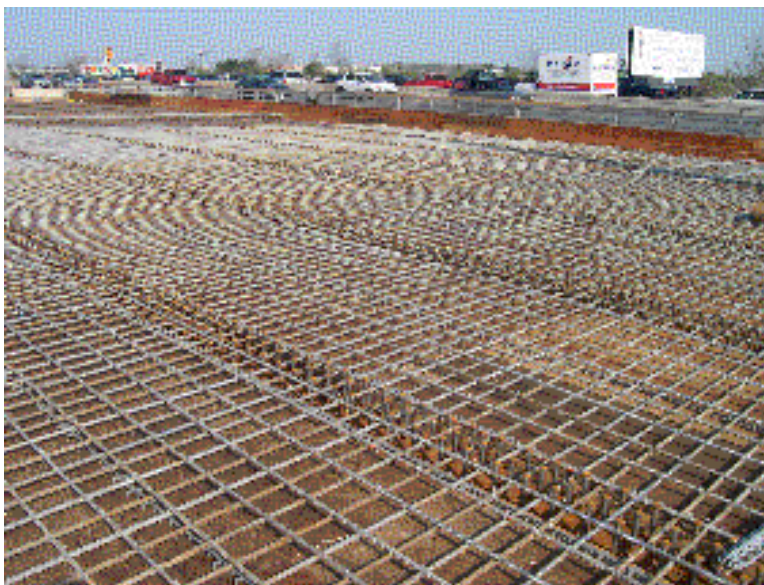
Figure 46. In-place galvanized reinforcement on the Frontage Road Bridge deck.
