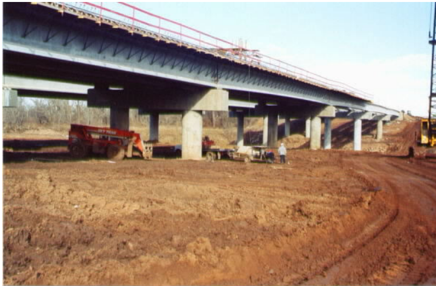
Figure 56. General view of the I-35 northbound bridge.
