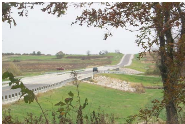
Figure 32. General view of the Route 6 bridges.
