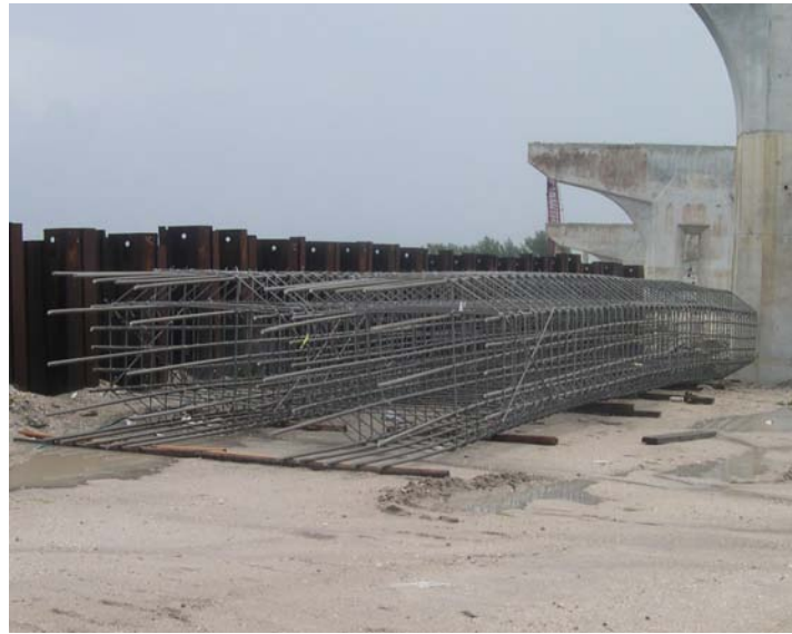
Figure 23. Photograph of 2201 ss reinforcement cage for the column of pier number 11.
