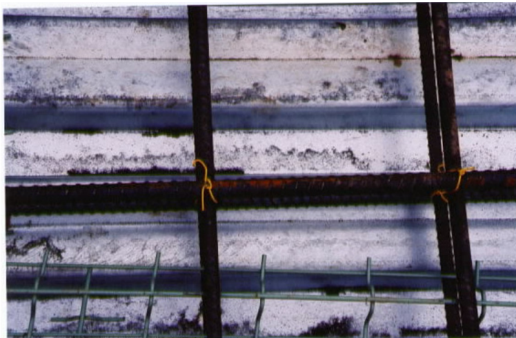
Figure 11 Closeup view of in-place reinforcing steel showing superficial corrosion.
