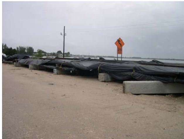
Figure 17. Photograph of stored MMFX-II reinforcing steel at the job site.
