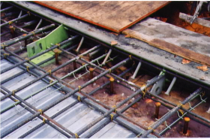
Figure 9. Closeup view of reinforcing steel, girder with shear studs, gusset plate, and forming for bulkhead.
