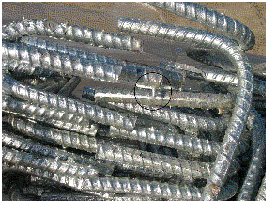
Figure 55. Galvanized layer disbonding and icicle on reinforcing bars. Examples of disbonding are also apparent.
