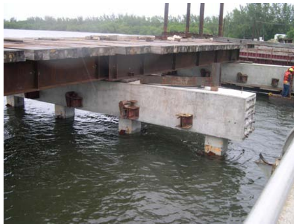
Figure 14. Photograph of substructure components prior to decking.
