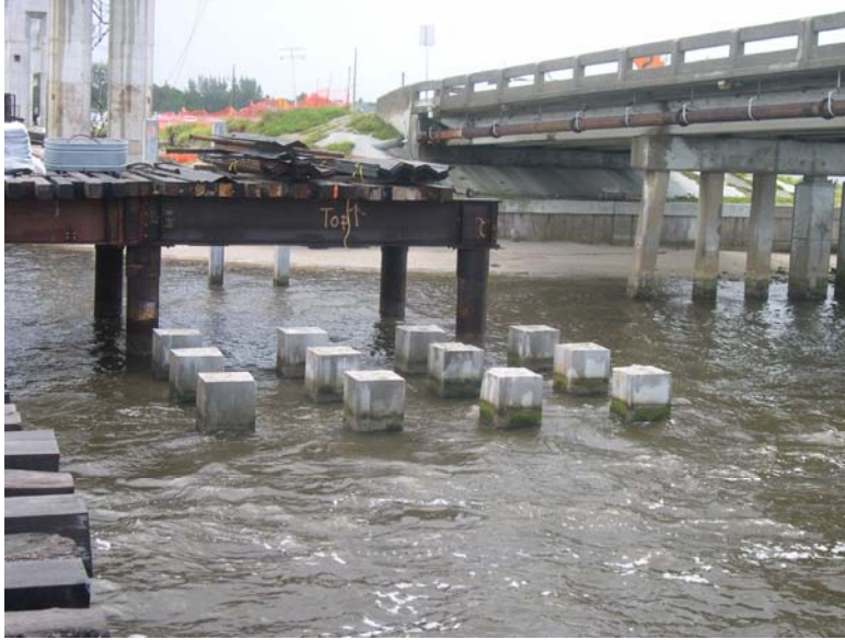
Figure 19. Photograph of driven, cut-off prestressed piles for pier 11.
