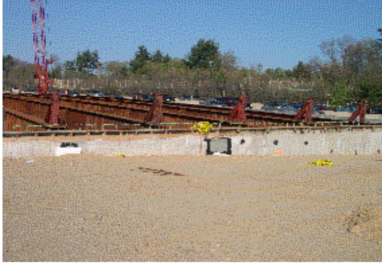
Figure 45. View of the in-place girders on the Brown Avenue Bridge. Note ECR extending from the top of the backwall.
