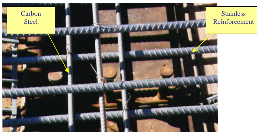
Figure 37. View showing carbon steel shear studs protruding through bottom mat of stainless steel reinforcement.
