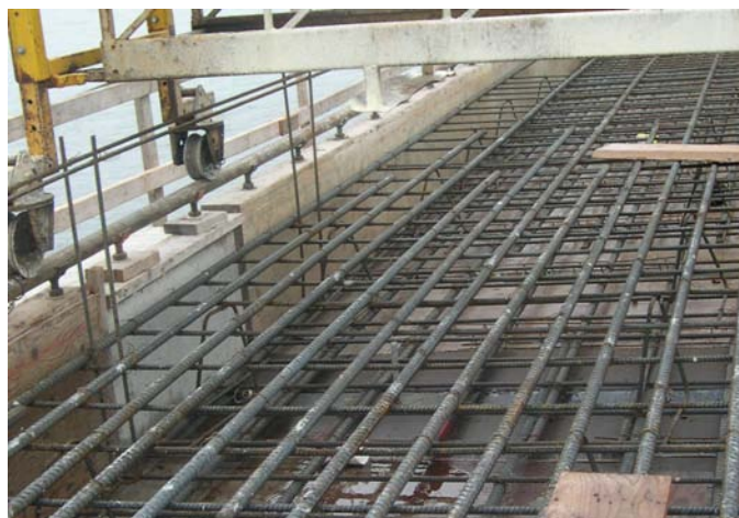
Figure 15. Photograph of MMFX-II deck steel in place.
