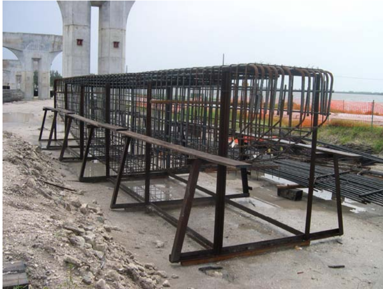
Figure 25. Photograph of the conventional bar reinforcement cage for a hammerhead column cap.
