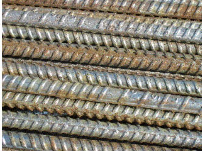
Figure 52. Deposits on galvanized reinforcing bars.
