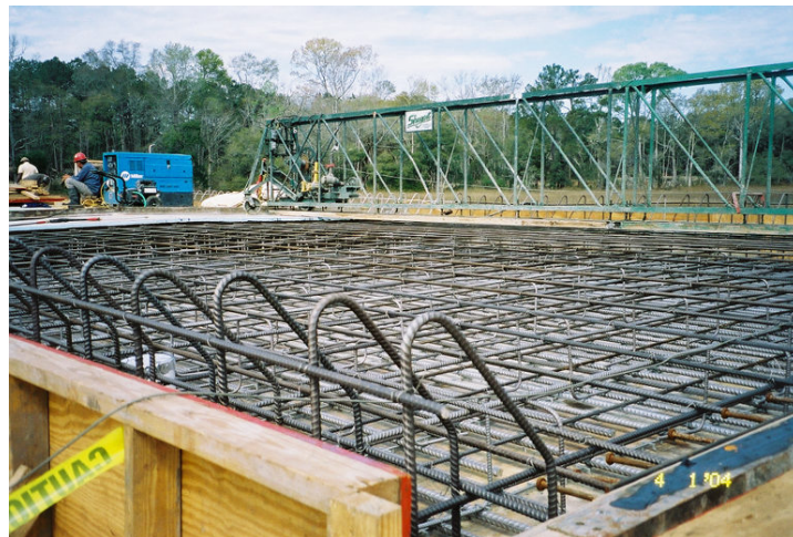
Figure 64. View of 2205 stainless steel placement in span 2.
