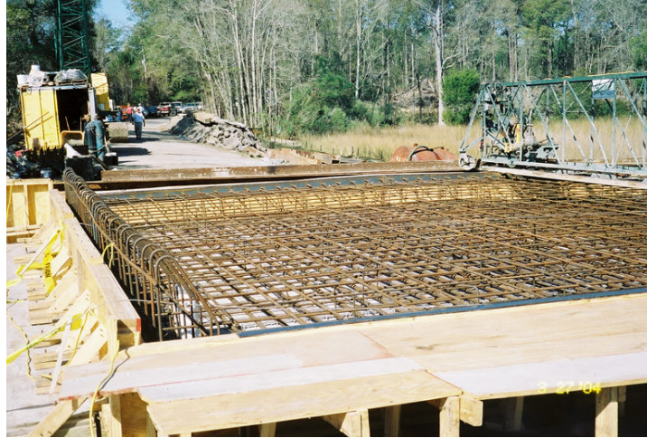
Figure 63. View of MMFX-II placement in span 5.
