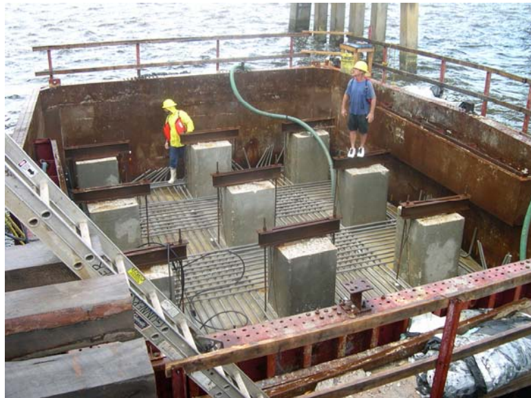
Figure 20. Photograph of formwork, piles, and reinforcement being placed in the footer of pier number 12.
