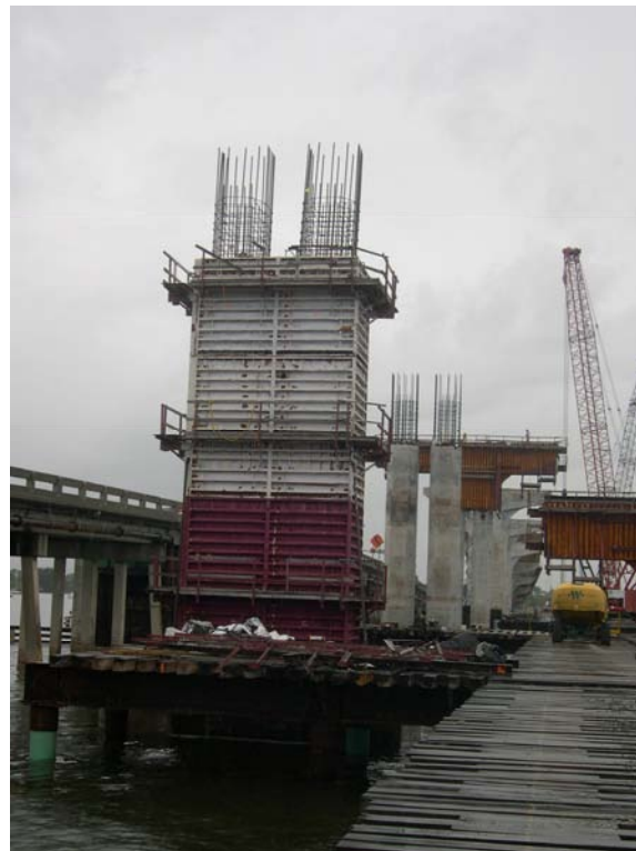
Figure 26. Photograph of pier number 11 column formwork and 2201 ss cage in place.
