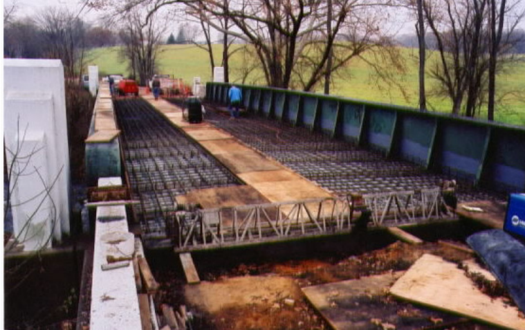
Figure 7. Photograph of the bridge deck with MMFX-II reinforcement in place.
