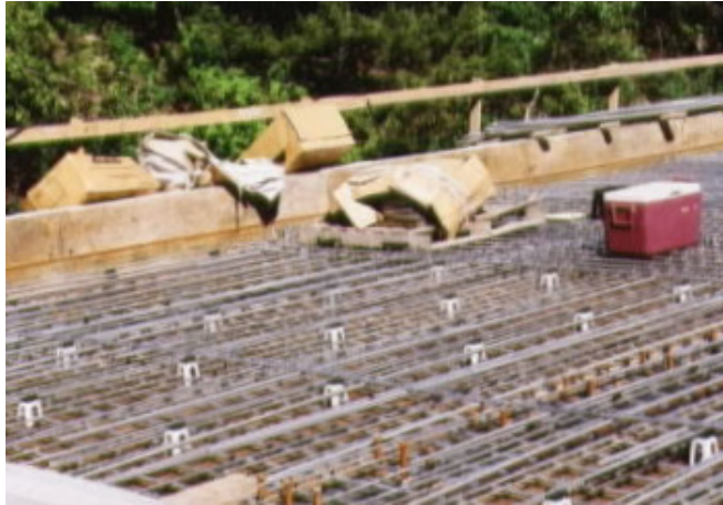
Figure 39. View showing cardboard packaged bent reinforcement details.
