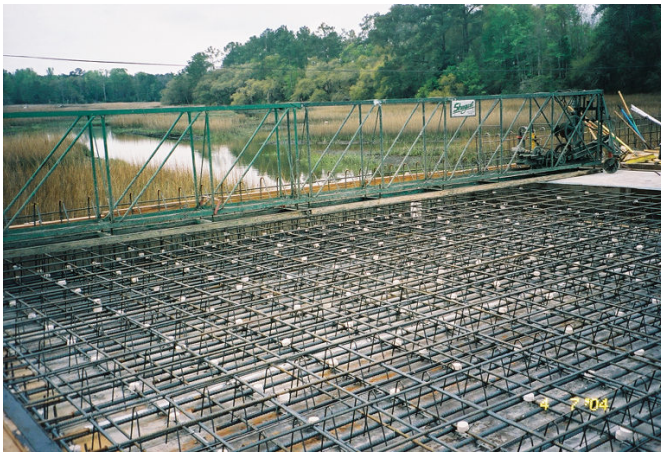
Figure 66. View of in-place black bars (span 1) along with discrete galvanic anodes.
