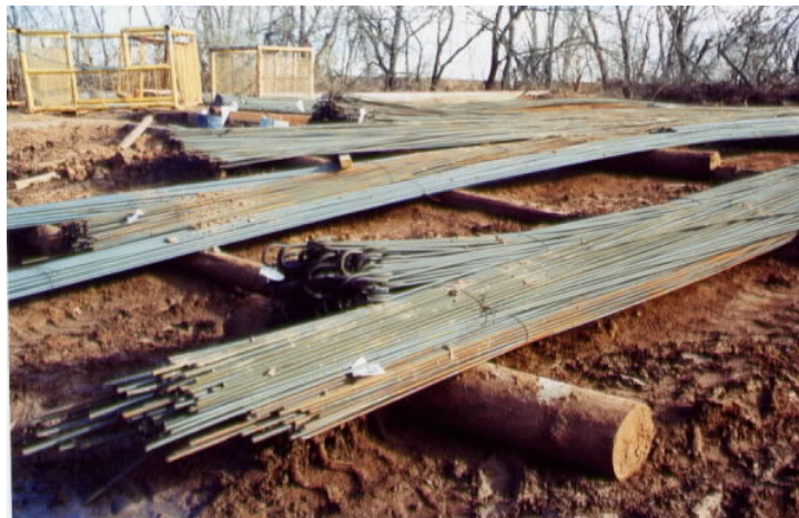
Figure 61. Closeup view of stored bars on timbers at job site.
