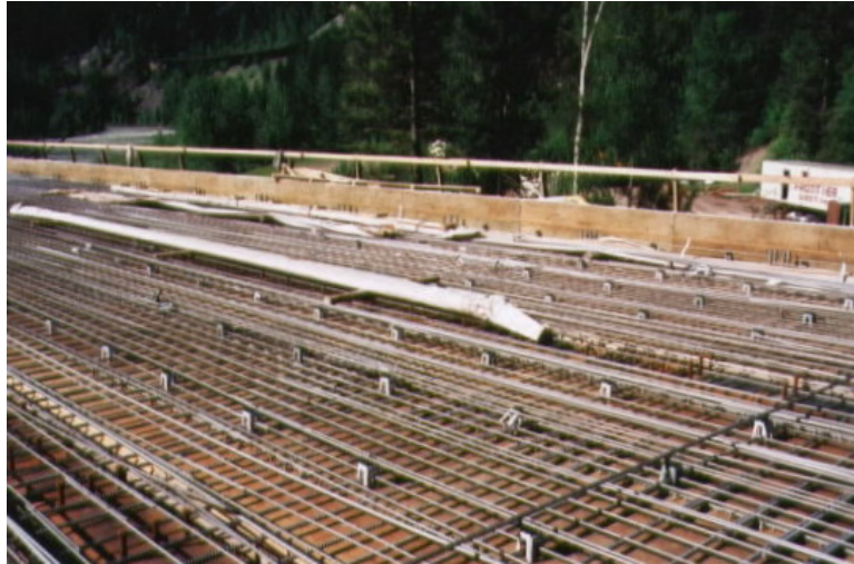
Figure 41. Array of plastic chairs to which bars from both mats are tied.
