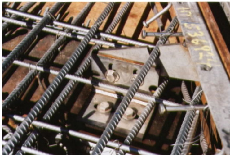
Figure 40. View of a guard angle adjacent to an expansion joint.
