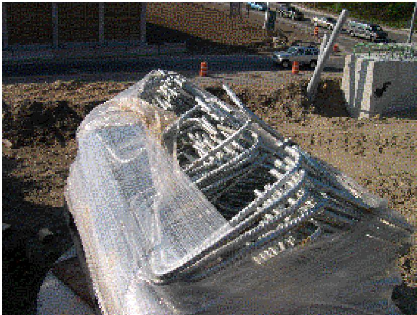
Figure 50. As-delivered galvanized bars at the Brown Avenue site after pulling back the plastic wrap.
