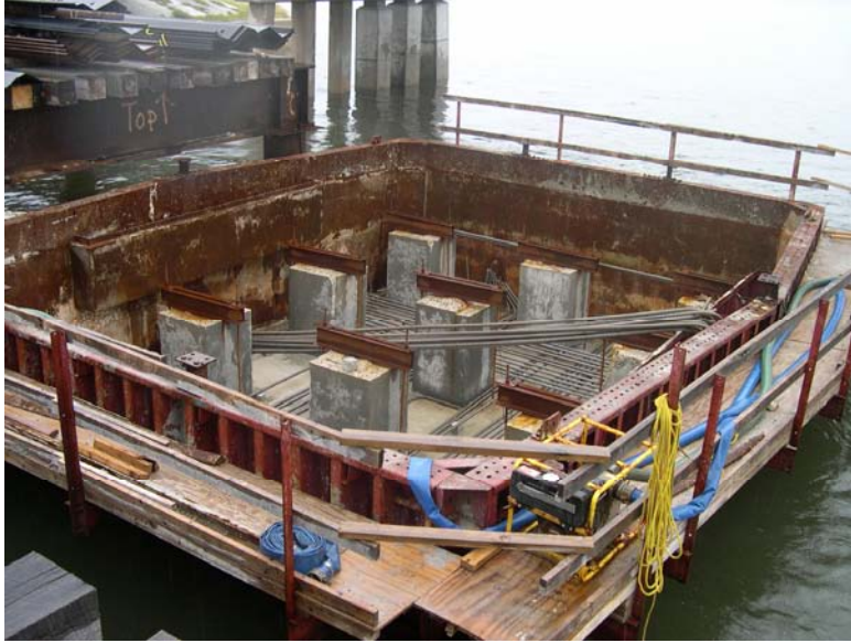
Figure 21. Photograph of formwork, piles, and reinforcement being placed in the footer of pier number 12.
