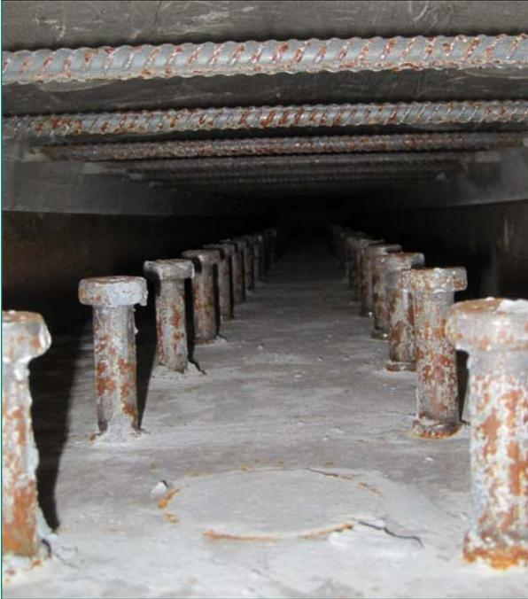
Figure 4. UHPC composite connection detail for concrete girders.
