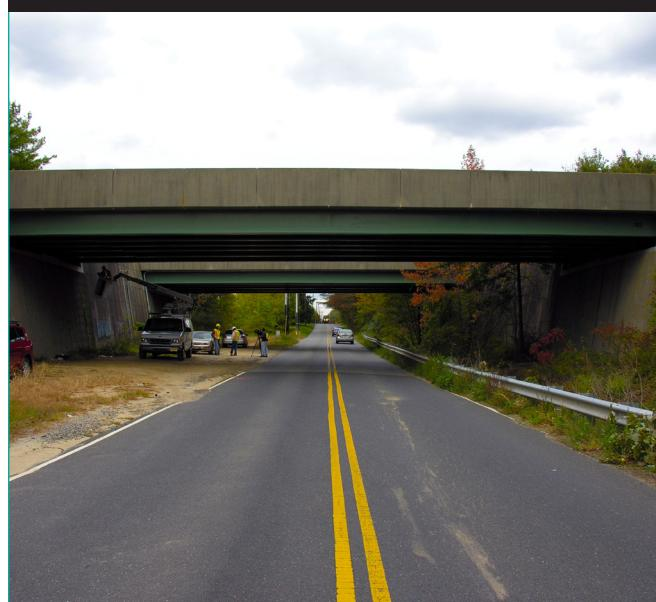
(LMC) overlay (nominal thickness of 1.25 inches) distributes live loads to the steel beams. An asphalt overlay was placed in 2010. The weather exposure and environmental conditions in central New Jersey represent a mixed-humid climate, as defined by the U.S. Department of Energy's climate zones. The bridge is exposed to frequent freeze-thaw cycles and application of deicing agents.
