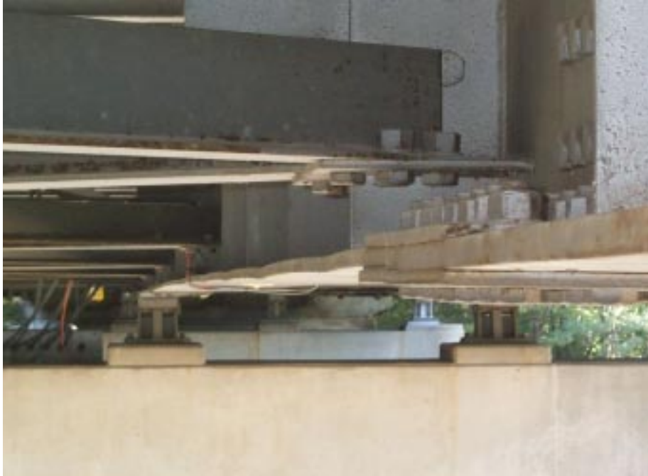
Figure 138. Flange distortion.
