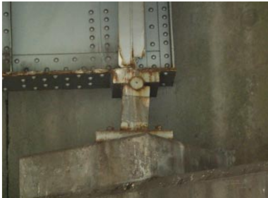
Figure 133. Rocker bearing rotation.
