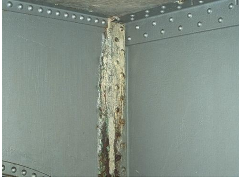
Figure 129. Typical efflorescence.
