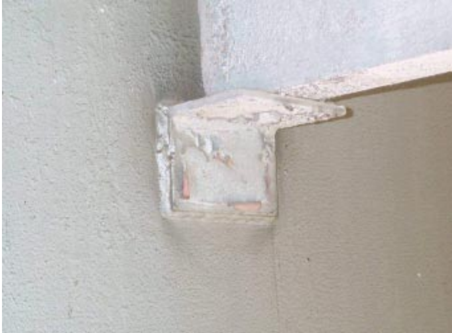
Figure 149. Typical utility bracket-to-web welded connection.
