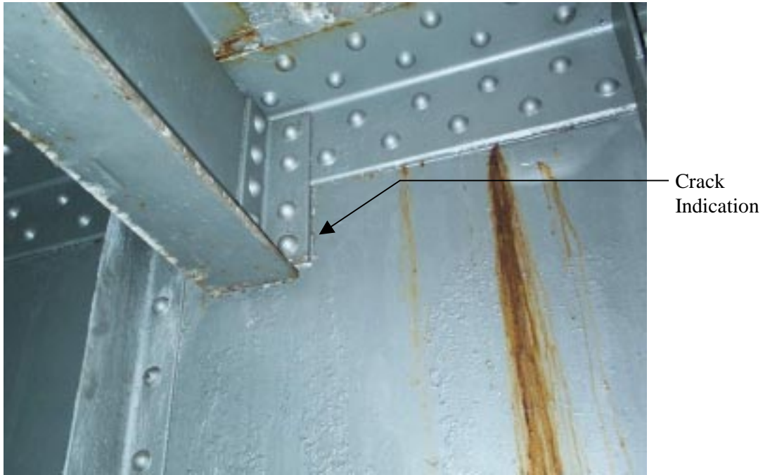
a. General location of implanted defect.
