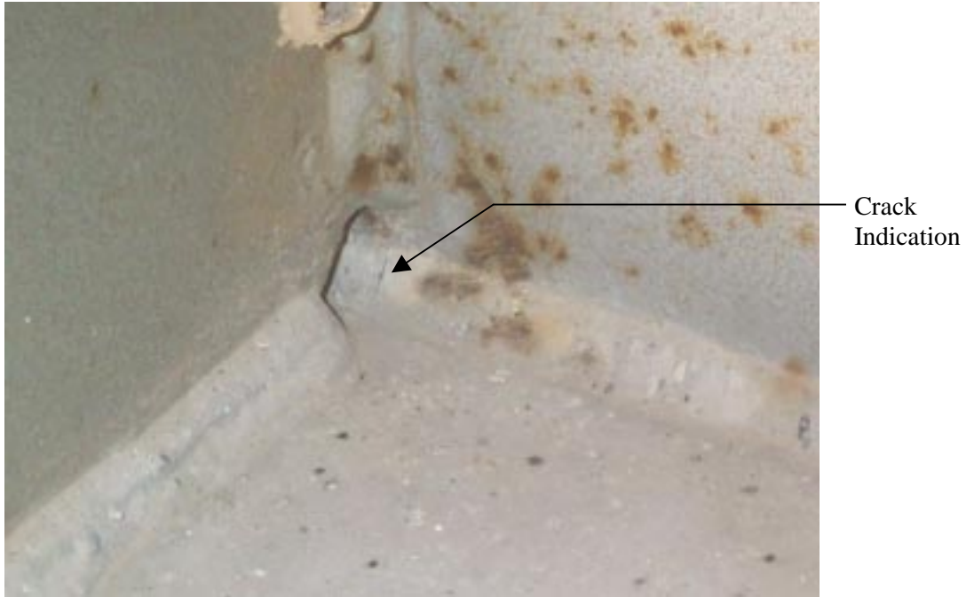
a. Web-to-flange connection.
