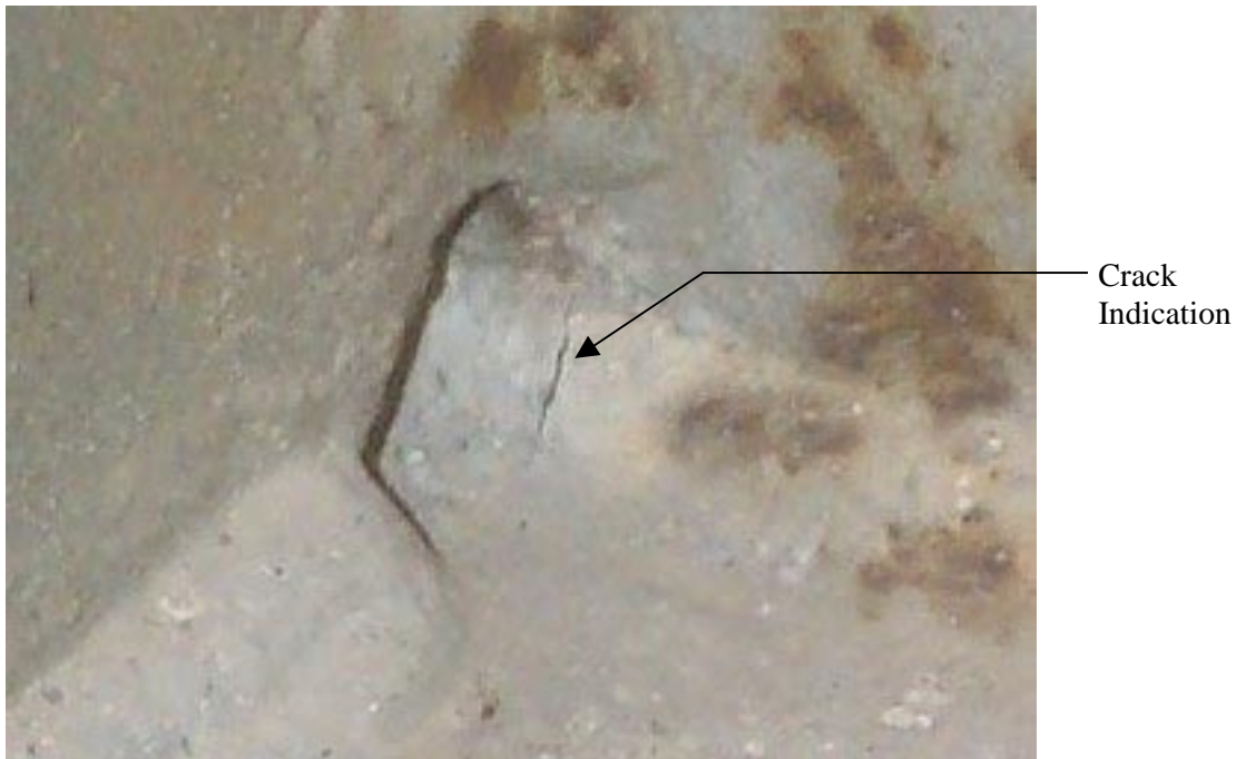
b. Crack indication enlarged for clarity.
