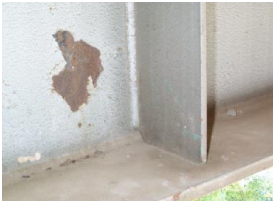
Figure 136. Paint failure on girder web.
