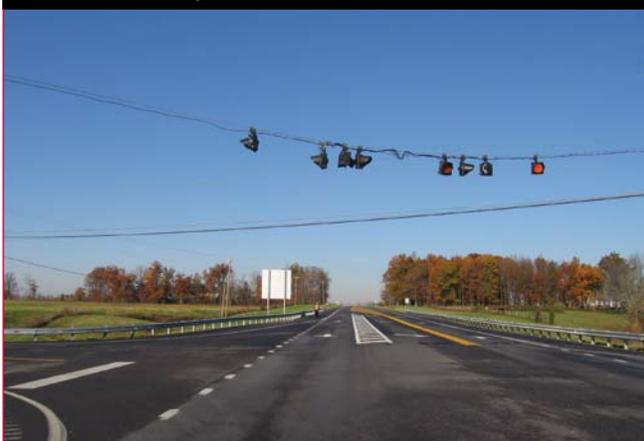
Furthermore, cross hatching in the median should also be provided for the lane-narrowing concept. Cross hatching will better define the presence and width of the median. In some of the deployments of the lane-narrowing concept, cross hatching was not used in the median. The treatment is much more conspicuous when cross hatching is used in the median (see figure 8 and figure 9).
