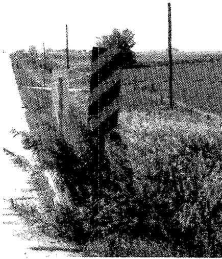
Hazard markers on low volume roads can be hidden by tall grass. This picture shows a marker at the end of a culvert that can be seen fairly well in daylight but will be partially hidden at night by the grass.
