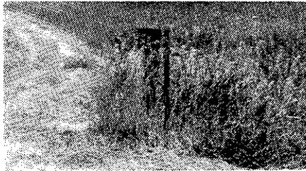
This photograph shows a hazard marker that will be completely hidden at night because the grass will shadow the marker from car headlights. Maintenance crews have mowed around the hazard marker. But they need to stop to trim around the marker or come back later to trim up.
