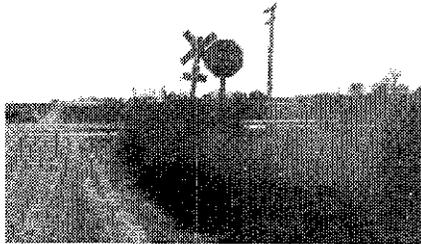
This is another rural railroad crossing. It has STOP signs in addition to the railroad crossbuck warning. But grass and weeds have been permitted to grow up in front of the STOP sign. Since the railroad tracks are on a sharp rise in the road, the grass and weeds prevent vehicle headlights from shining on the STOP sign at night. This vegetation needs to be cut immediately.
