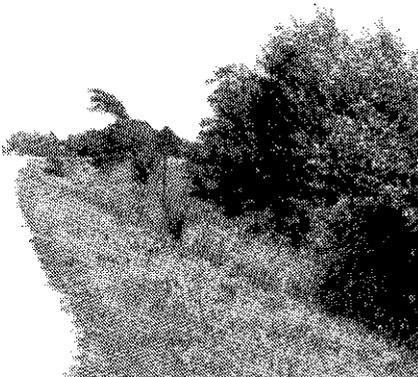
This photograph shows a rural roadside that has been well maintained only on the foreslope into the ditch. Brush in the ditch and on the back-slope is beginning to block the STOP AHEAD sign. Soon it will block the driver's view of the STOP sign in the far distance. If these young trees are allowed to continue growing, they will become hazards.
