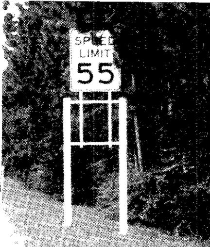
Here tree limbs that have been trimmed back in previous years are beginning to grow back in front of the sign. Maintenance patrols need to look for trees and brush that block the view of signs or other traffic control devices.
