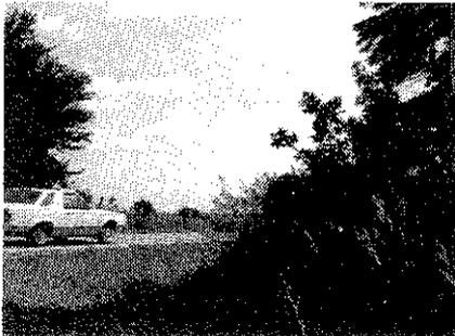
This intersection has tall grass and weeds in the ditch and a backslope area that creates a hazard. There is a STOP sign, but after stopping, a driver must pull out onto the edge of the main road to see around the weeds. Vegetation in the ditches has to be kept low enough to allow good sight distance at intersections.
