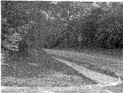
At this same location, street maintenance crews flattened the slope from the sidewalk to the property line and cut the trees and bushes. A landscape architect for the city placed low-growing plants on the yard slope to reduce future maintenance. This method greatly improved drivers' visibility of the conflicting traffic.
