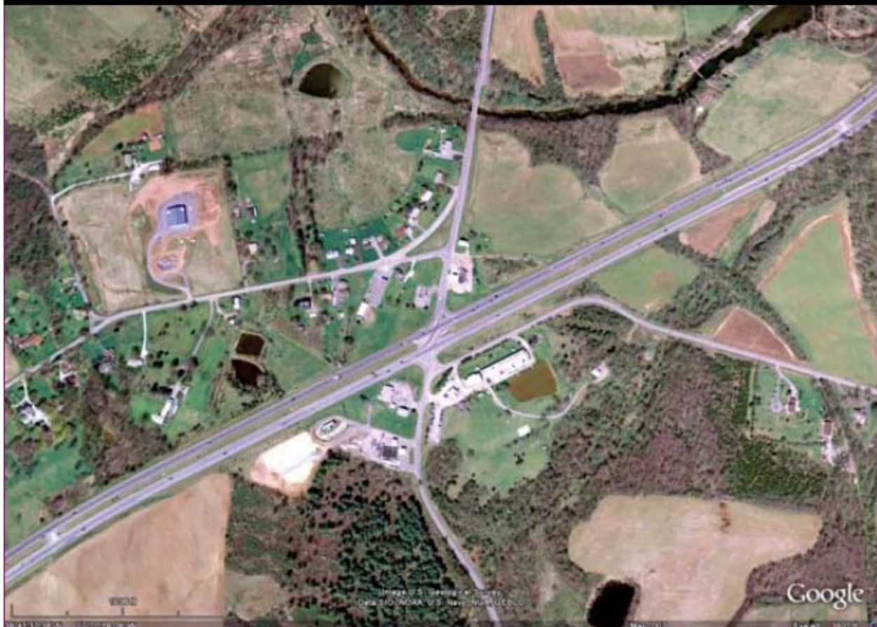
Figure 1. RCUT intersection observed in this study.
