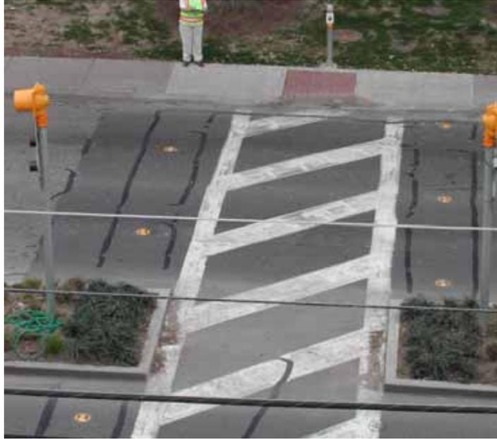
**Figure 10-11. Photo. Working example of in-roadway warning lights with pedestrian pushbutton in Austin, TX.**
