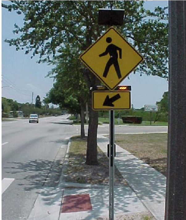
Figure 1. RRFB with two forward-facing LED flashers and a side-mounted LED flasher.
