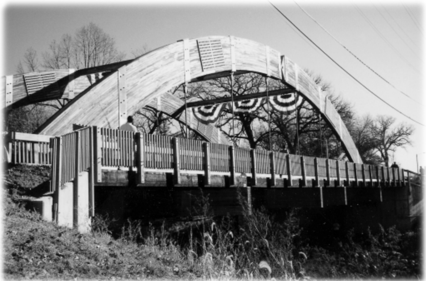
This glulam three-pin arch vehicular bridge, located in Nebraska, was funded by FHWA through ISTEA's Timber Bridge Demonstration Program.
