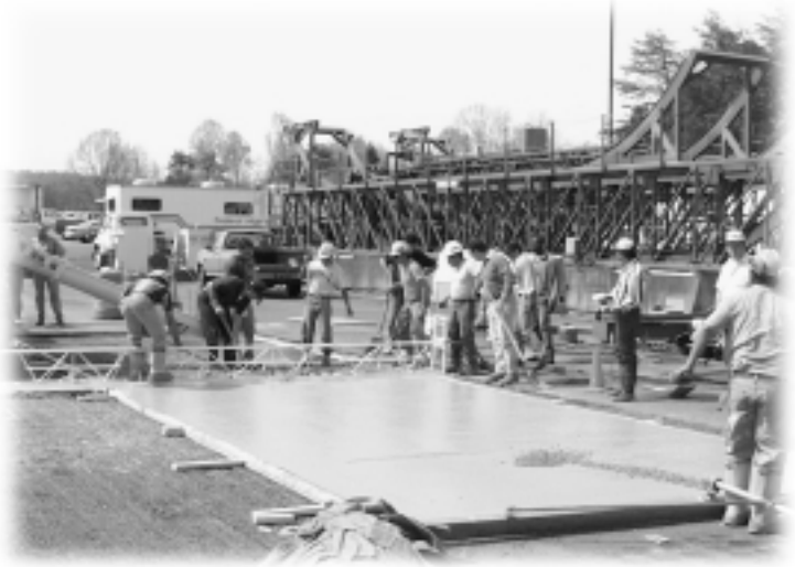
UTW test sections were constructed in May 1998 at TFHRC. Loading began soon afterward using the ALF machines. (ALF machine pictured in background.)
