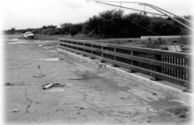
Figure 2 — Bridge rail and pick up after the crash test.
