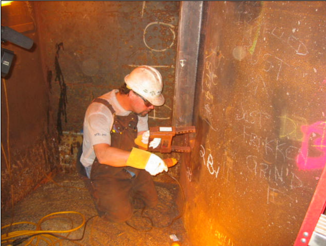
Figure 16: MTE inspector Mark Vasallo performing magnetic particle examination on pile head connection weld 2-B in Pier Footing Structure E4W.
