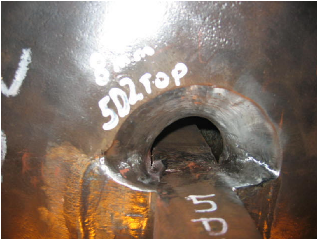
Figure 12: Top of pile connection plate weld at location 5D after grinding magnetic particle indications at tab removal sites.
