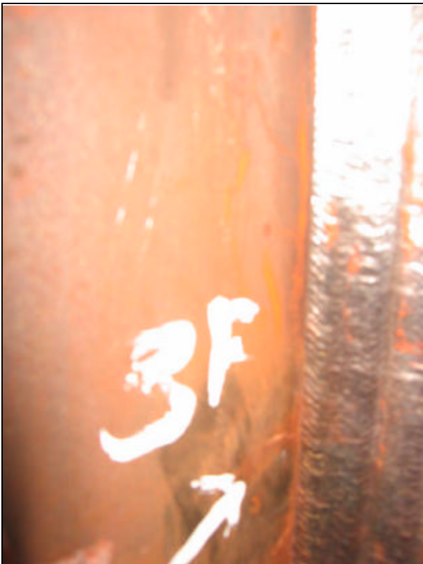
Figure 15: Magnetic particle indication at pile connection plate weld 3F in connection plate. Indication removed by light grinding, no flaw detected.
