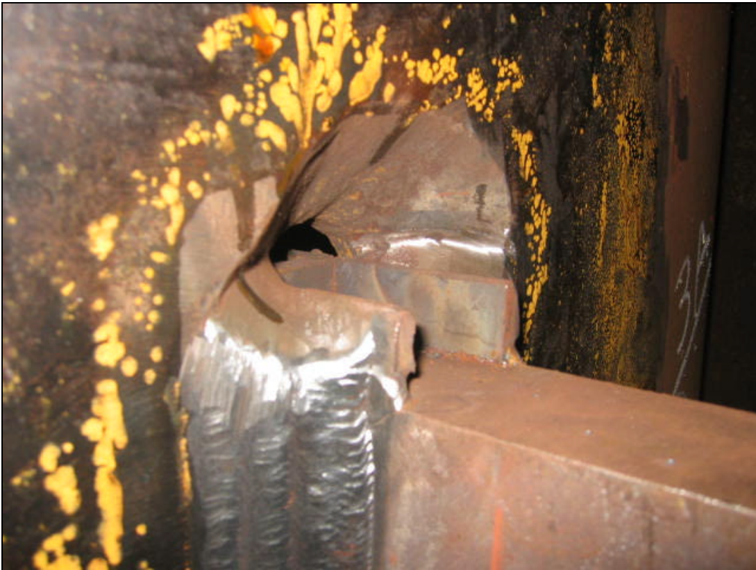
Figure 8: Weld tabs in place at top of pile connection plate weld.
