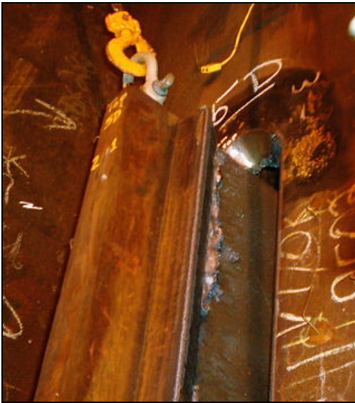
Figure 17: Removal of weld sample 5D.
