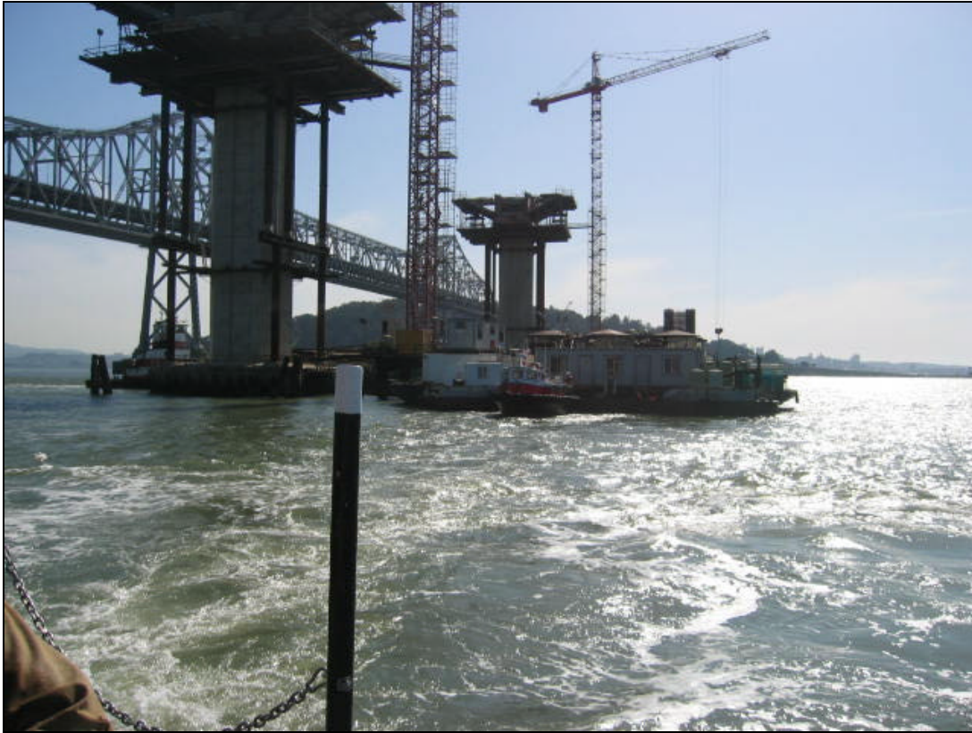
Figure 1: Pier footing at E4W
