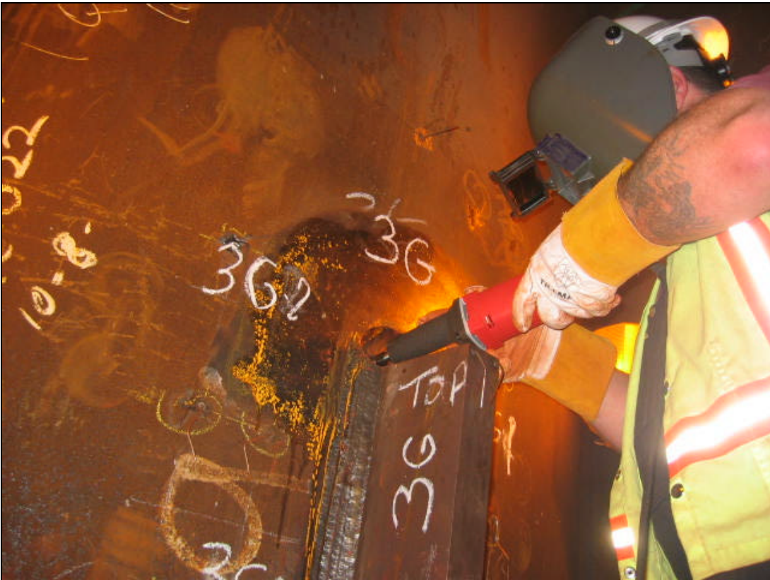
Figure 10: Grinding by MTE inspector Mike Virgillio to investigate magnetic particle indications at tab removal sites at location 3G.
