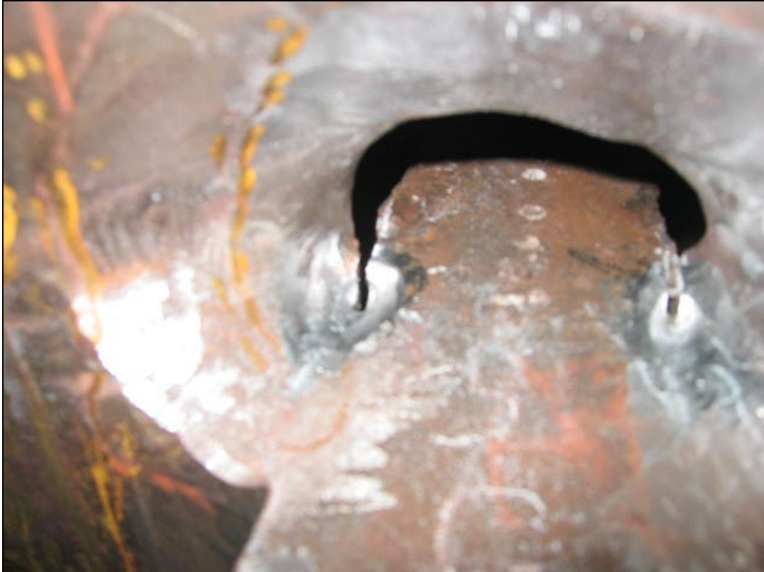
Figure 11: Tab removal site at location 3G after exploratory grinding. Magnetic particle indications no longer appear.
