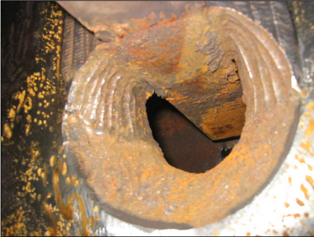
Figure 9: Bottom of pile connection plate weld, after weld tab removal, before grinding.
