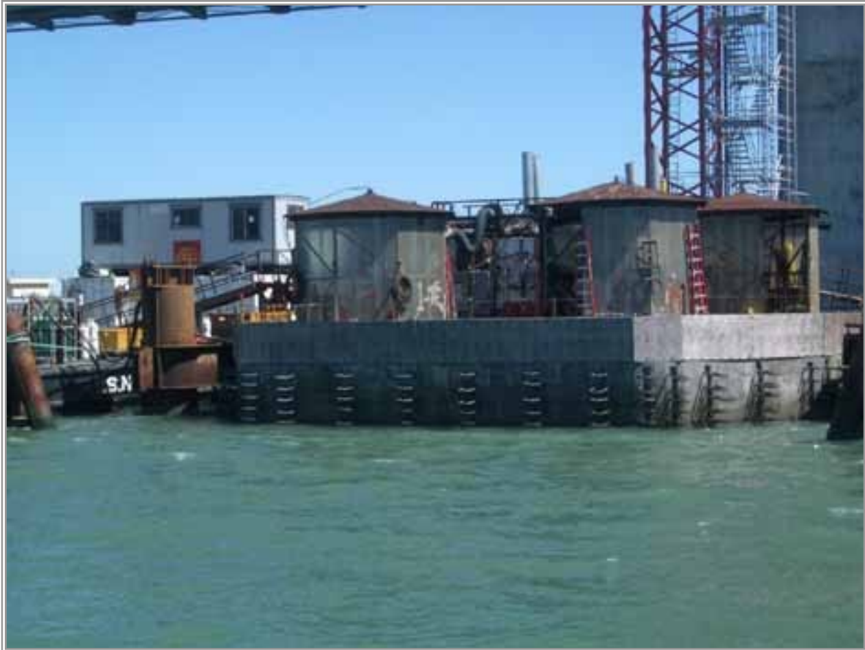
Pier E5W Foundation Box
