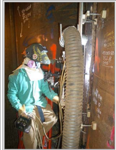
Welding Intermediate FCAW Weld Pass 9, PJP 1A1
