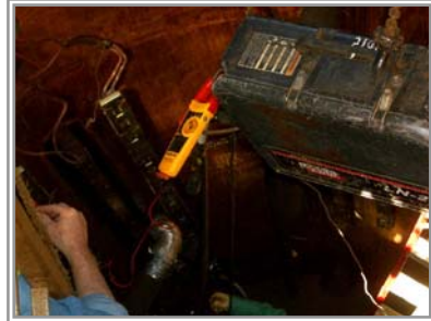
QC Monitoring Weld Parameters
