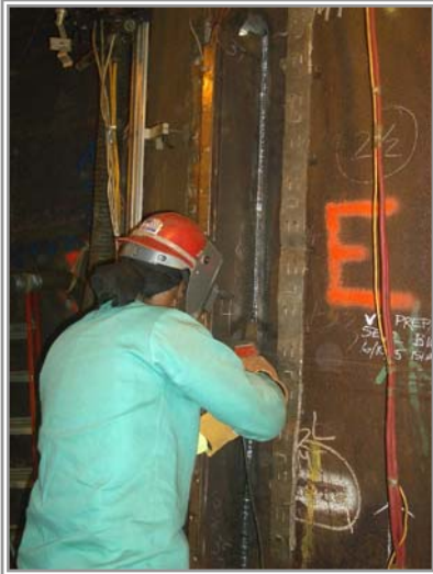
MT Root Pass Pile 5, Joint E1
