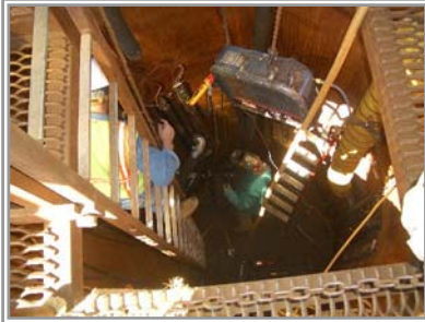
Typical Welding Machine Set Up Inside Pile, Joints 3 & 4
