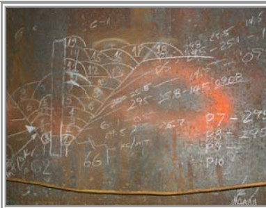
Record of Weld Pass Progression on Pile Wall, PJP 6G1 & 6G2
