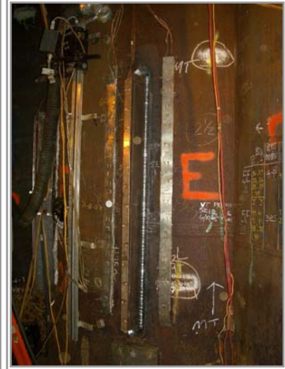
Typical PPJ Pile 5, Joint E1
