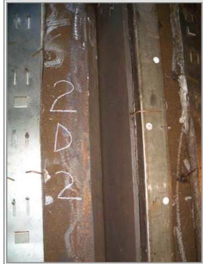
Typical Joint Preparation PJP 2D2
