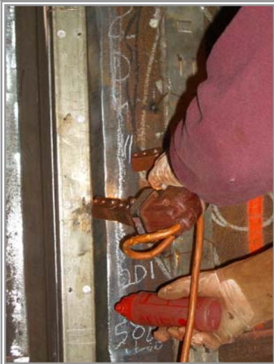
QC MT Tack Welds PJP 2D1
