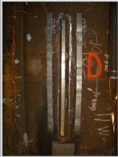
PJP 2D1 Tack Welded in Preparation for Root Pass
