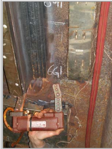
MT Final Cover Pass While Hot PJP 6G1
