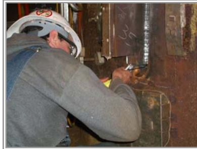
QC Inspecting PJP Access Area, Pile 5, Joint E1
