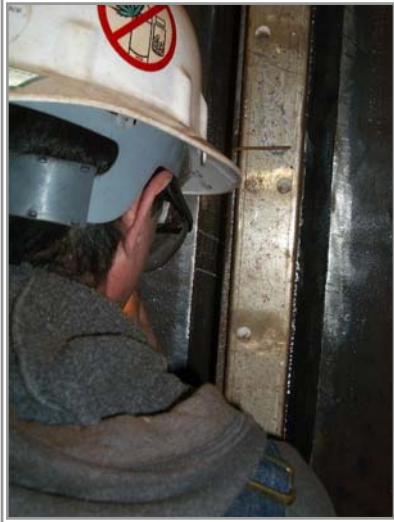
QC Inspecting Joint Fitup Prior to Root Pass, 5E1 & 5E2
