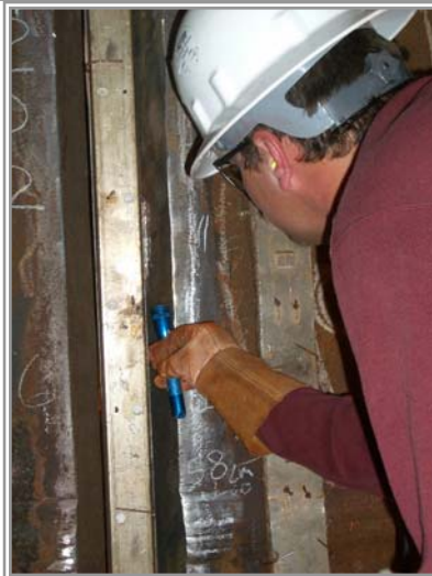
QC Visual Inspection of PJP 2D1 Prior to Welding Root Pass
