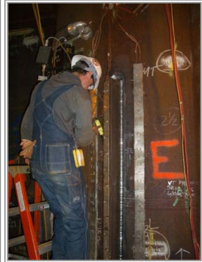
QC Inspecting Weld Pass Joint 5E1
