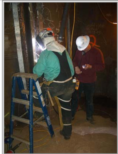
Welding Root Pass, PJP 2D1 Timing Travel Speed
