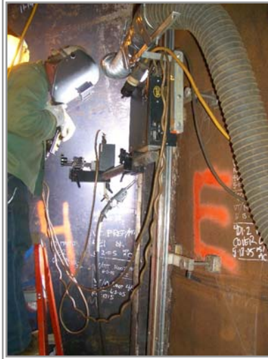
Welding Root Pass Pile 5, Joint E2
