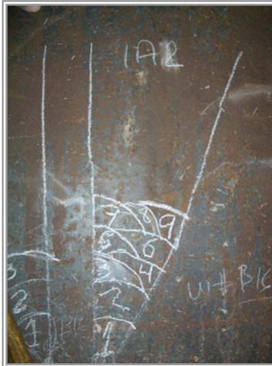
Record of Weld Pass Progression on Pile Wall, PJP 1A1 & 1A2
