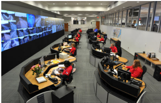
Figure 2 NCDOT ITS Operations Center
