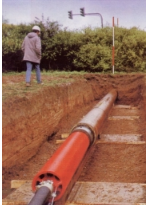
Figure 14. Pipe Ramming Entry Pit. (20)
