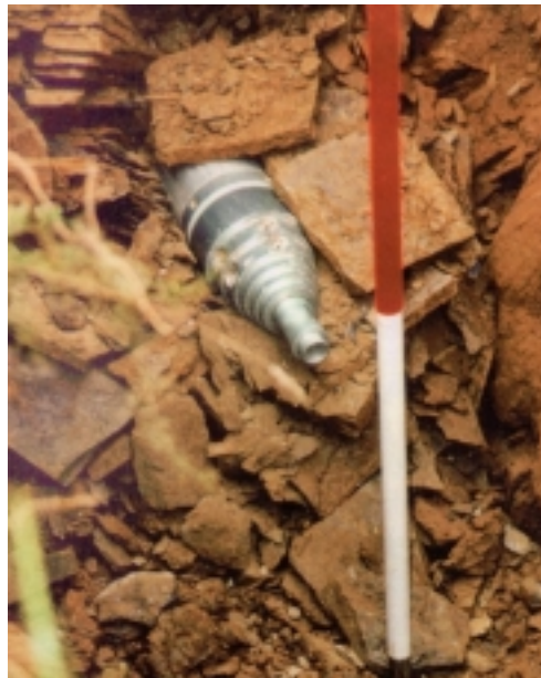
Figure 15. Stepped Cone Impact Moling Head Emerging at the Reception Pit. (20)
