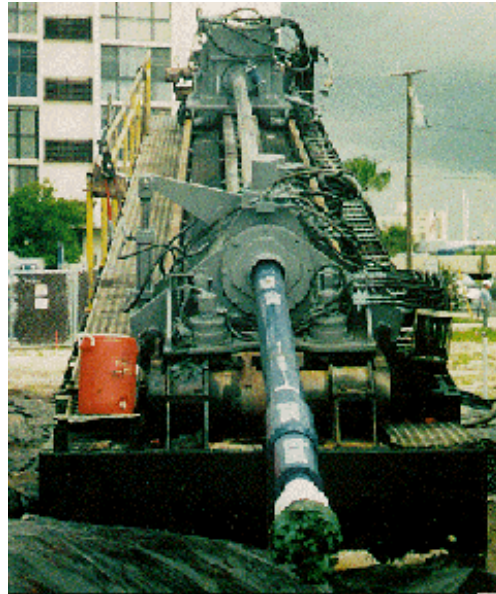
Figure 3. Surface-Launched HDD Rig (Courtesy of Purdue University).
