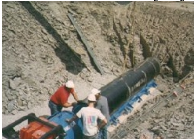
Figure 7. Track-Type Auger Boring Operation (Courtesy of Purdue University).
