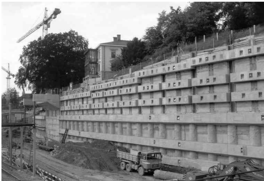
Figure 1. Photo. Retaining wall of the train station Stadelhofen in Zurich, Switzerland.
