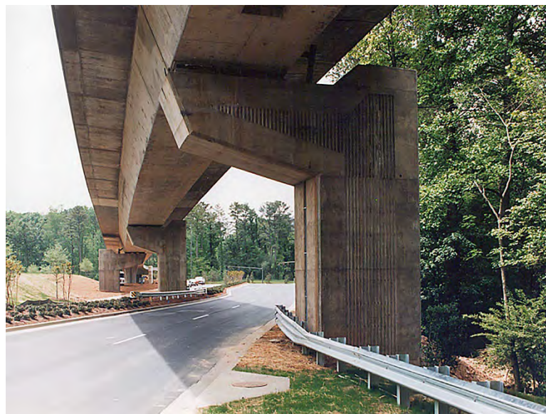
Figure 1.6 Hammerhead Piers (T-Piers), Straddle Bents, and Integral T-Piers
