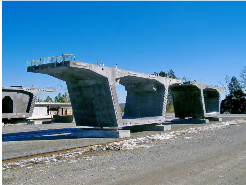
Figure 8.2 Precast Concrete Segments for the Foothills Parkway Bridge No. 2
