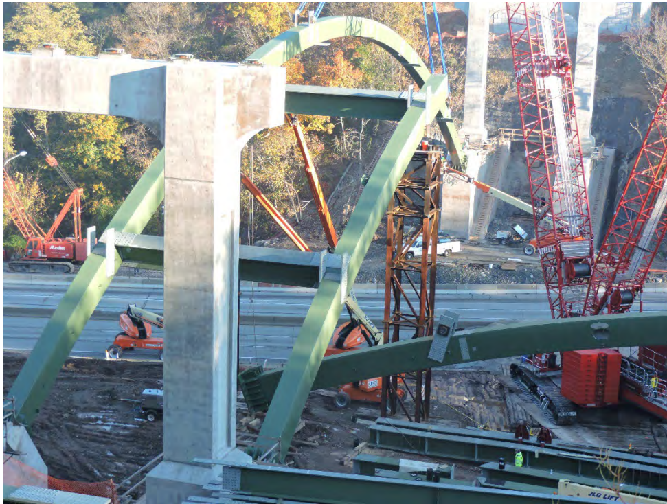
Figure 14.4 Erection of the Arch Rib of the Greenfield Bridge in the City of Pittsburgh Using Temporary Supports
