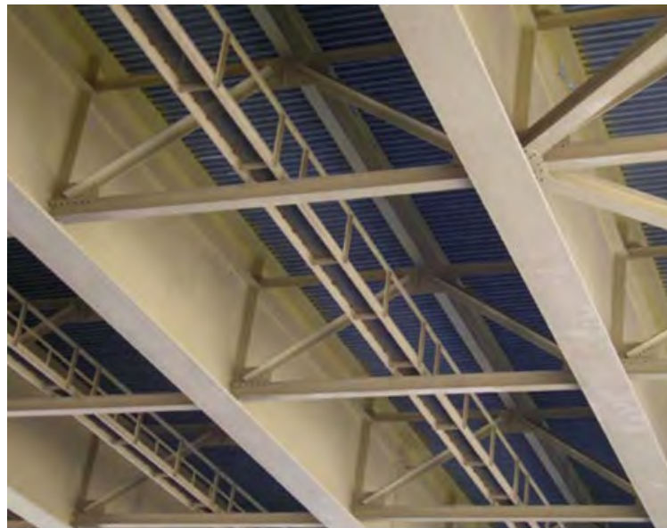
Figure 11.1 Girder-Substringer System
