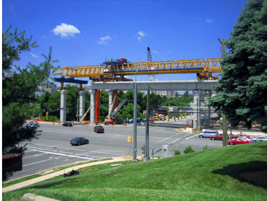
Figure 8.6 Span-by-Span Construction with Overhead Gantry on the Phase 1 Dulles Corridor Metrorail Project
