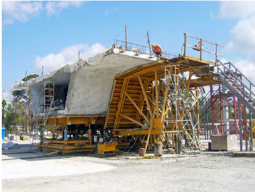
Figure 8.10 Casting Machine for the I-95/I-295 Ramp in Jacksonville, Fla.
