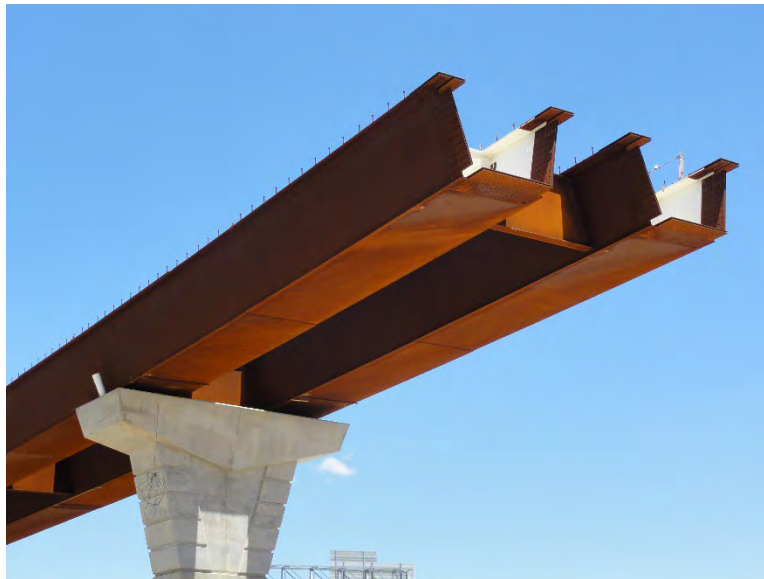
Figure 12.1 Dual Steel Trapezoidal Box Girders
