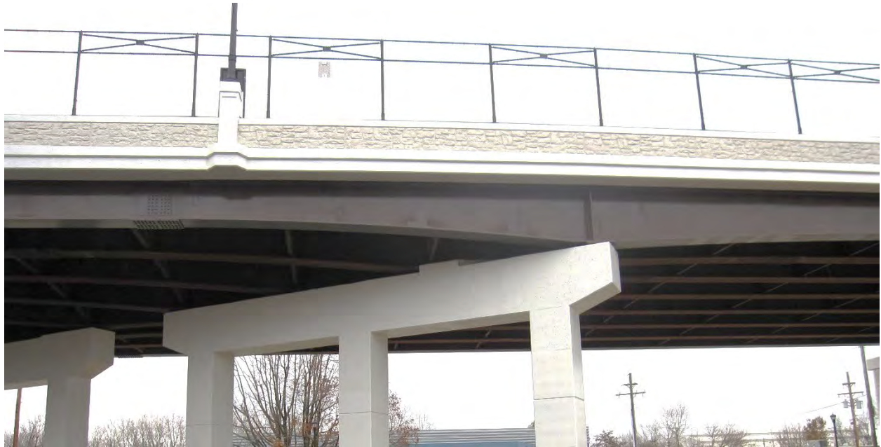
Figure 10.25 Application of Parabolic Variable Depth Girders
