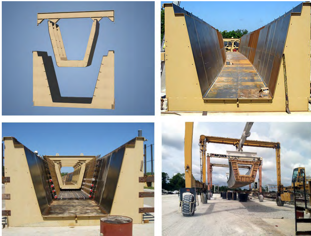
Figure 9.2 Curved U-Girder Fabrication
