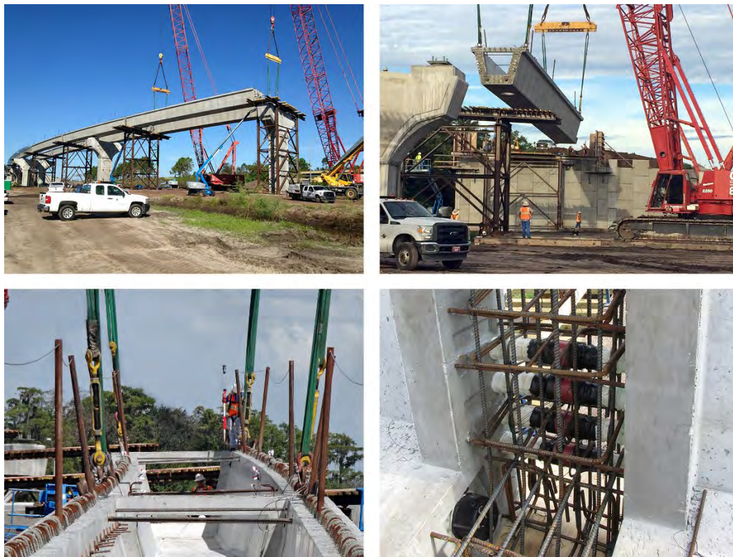
Figure 9.3 Curved U-Girder Field Assembly
