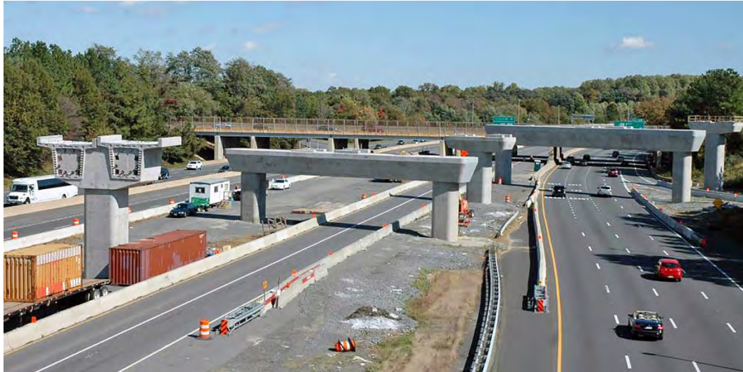
Figure 1.6 Hammerhead Piers (T-Piers), Straddle Bents, and Integral T-Piers
