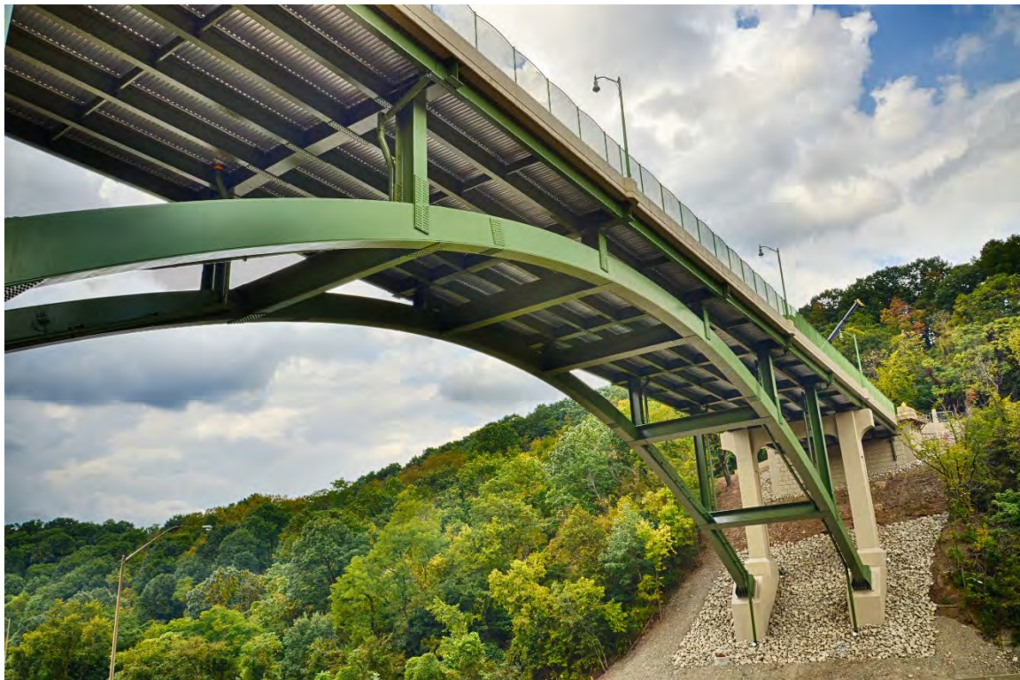
Figure 14.1 Greenfield Bridge in the City of Pittsburgh, an Open-Spandrel Deck Arch Structure Completed in 2017
