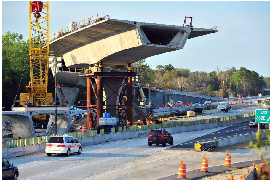
Figure 8.4 I-95/I-295 Ramp Balanced Cantilever Construction, Jacksonville, Fla.
