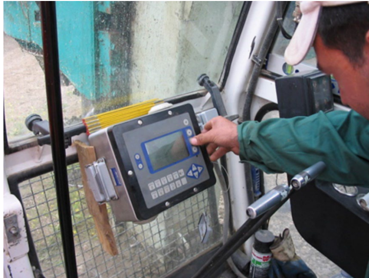
Figure 2-5 Automated Monitoring During CFA Pile Construction (from FHWA GEC 8, Brown, et al, 2007)
