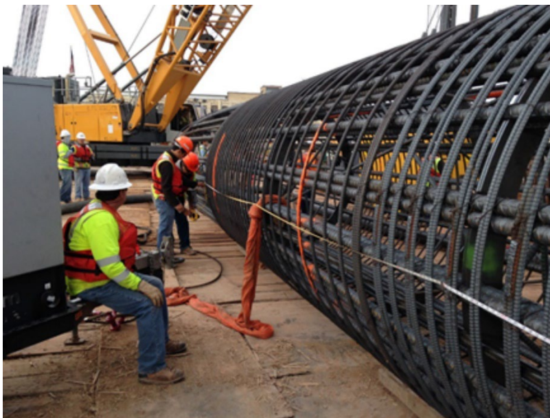
Figure 3.1 Evaluation of steel reinforcement for a drilled shaft (photo by the authors).
