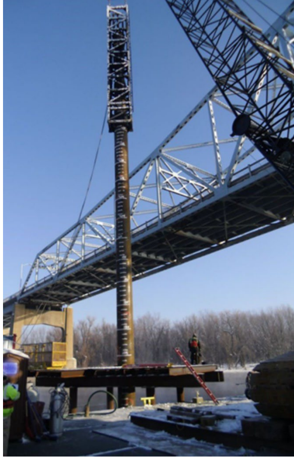
Figure 2-4 Test Pile Installation to Develop Driving Criteria (photo by the authors)
