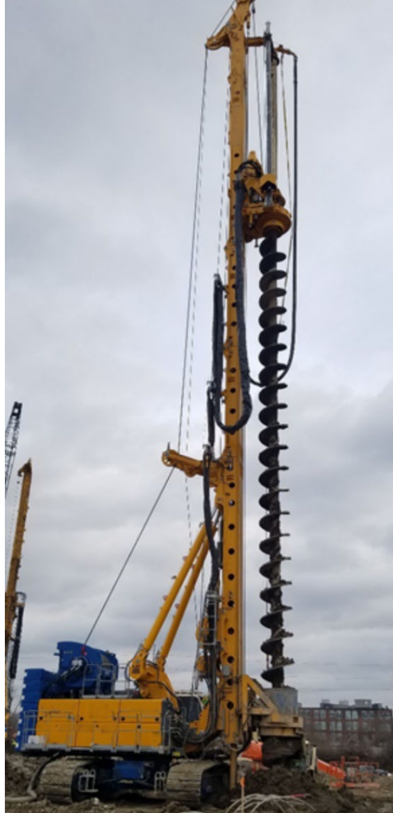
Figure 7-1 CFA Piling Rig (photo by authors)
