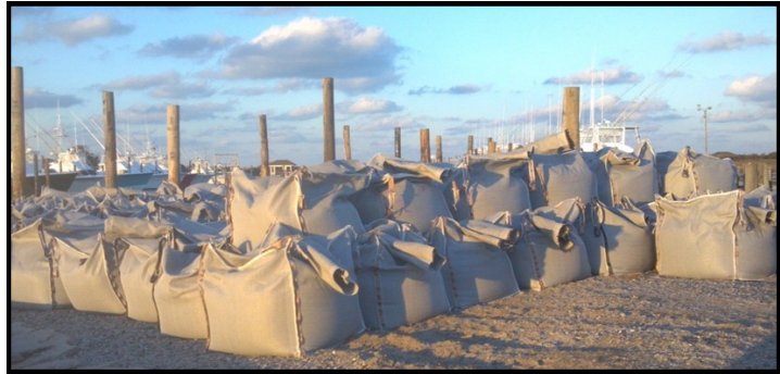
Figure 11—Geotextile Sand Bag Stockpile (4'x4'x4' cubes)
