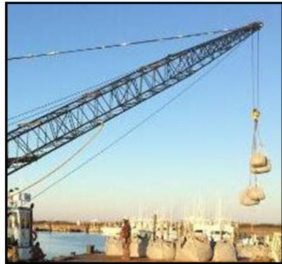
Figure 20—Contractor lifting the Sand Bags to place at Bent
