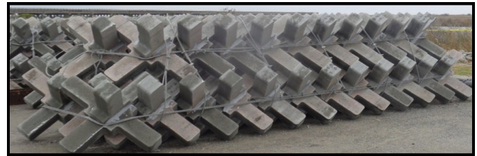
Figure 16 - Stainless Steel Cable & Hardware Binding
