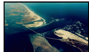
Figure 2—Aerial photo of Bonner Bridge
