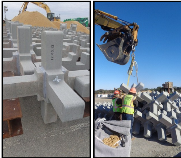
Figure 15—A-jacks® Assembly Area and Stockpile
