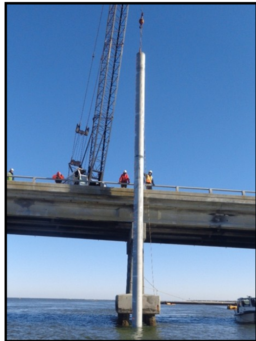
Figure 13—Bonner Bridge Test Pile #2
