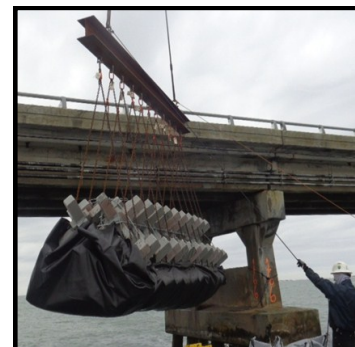
Figure 18—Geotextile Filter Applied to A-jack® Logs
