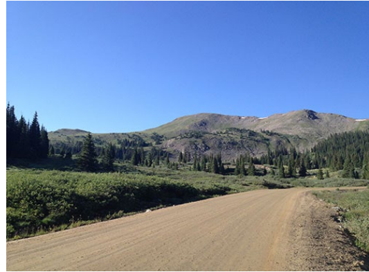
Figure 1: Before Construction, Existing Road at Western Limit. Image courtesy of FHWA.
