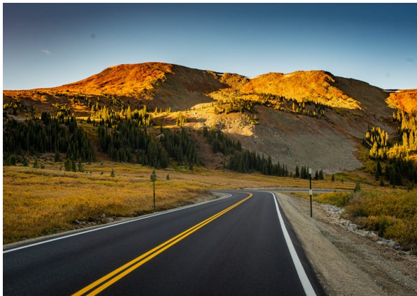
Figure 2: Completed Road below Summit. Image courtesy of FHWA.
