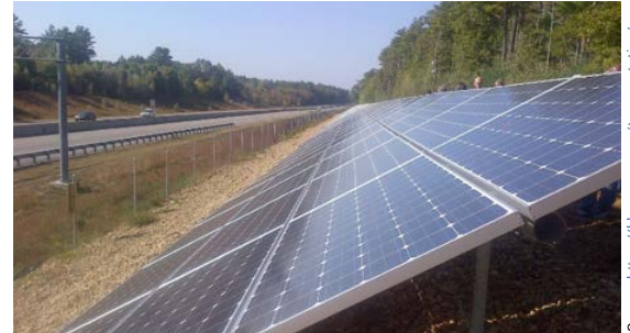
MassDOT solar project along Route 44.
