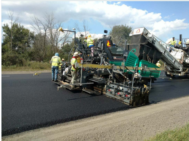
An infrared camera, mounted above the paver screed, detects significant temperature differentials in the mat. Photo: ©Tim Murphy.
