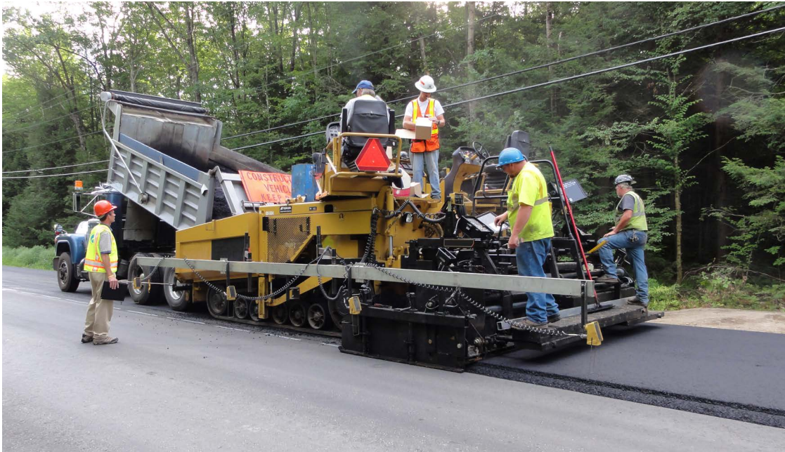
Here, a crew uses a paving machine to place and finish an asphalt concrete surface layer. Pavement designers can use FHWA's catalog to facilitate planning, budgeting, and design checks for new pavements. Photo: ©Shreenath Rao, Applied Research Associates, Inc.
