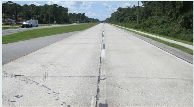
Category #1. No structural deterioration. Requires functional preservation.
