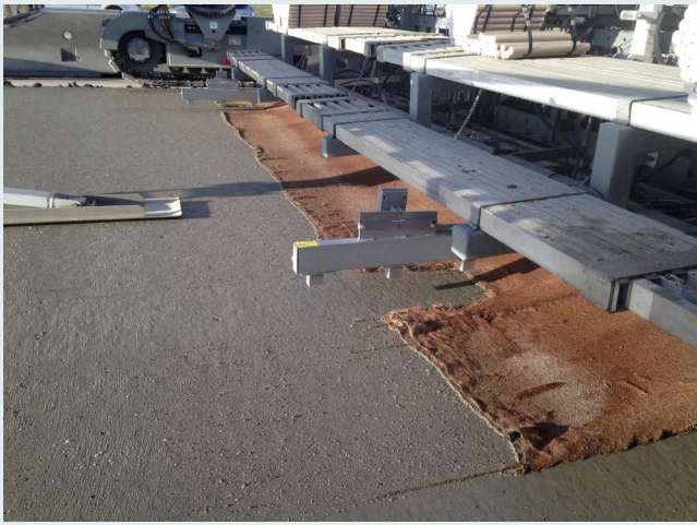
Real-time smoothness systems like the one shown here installed on the back of a concrete paver are the topic of one of the videos in the Concrete Clips series. Photo: ©Gary Fick, Transtec Group, Inc.
