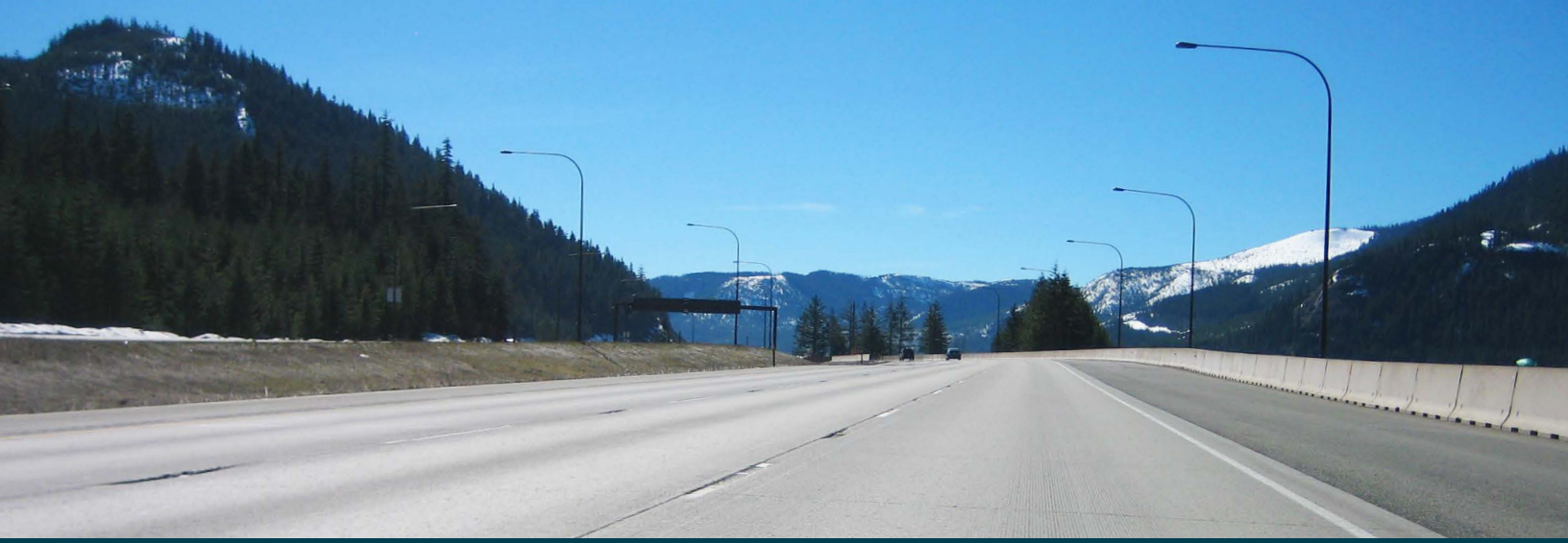
FHWA efforts help State highway agencies build concrete pavement roads that last longer. Photo: ©APTech.
