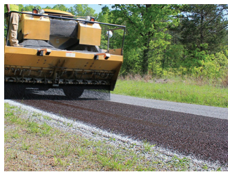
Slurry Pavers, Inc. Figure 1. Chip sealing
